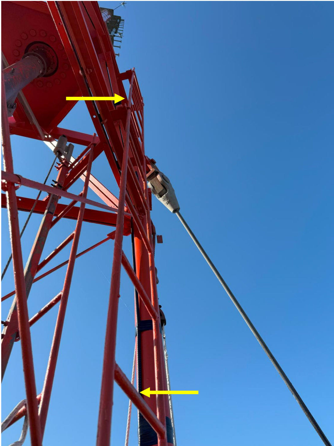
WLPB TV 990' Tower Inspection August 18 th , 2025
