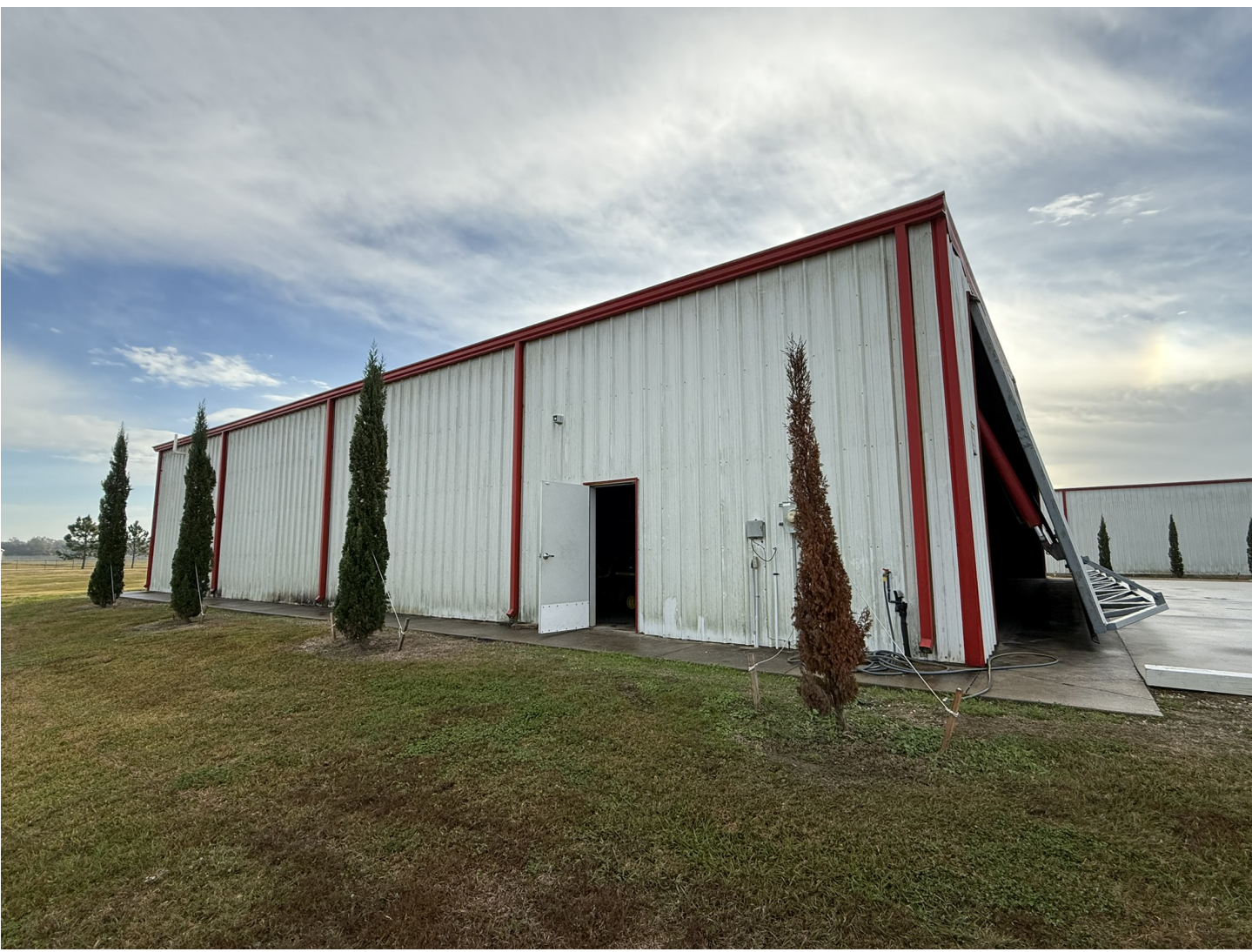
PHOTO OF NORTH ELEVATION
