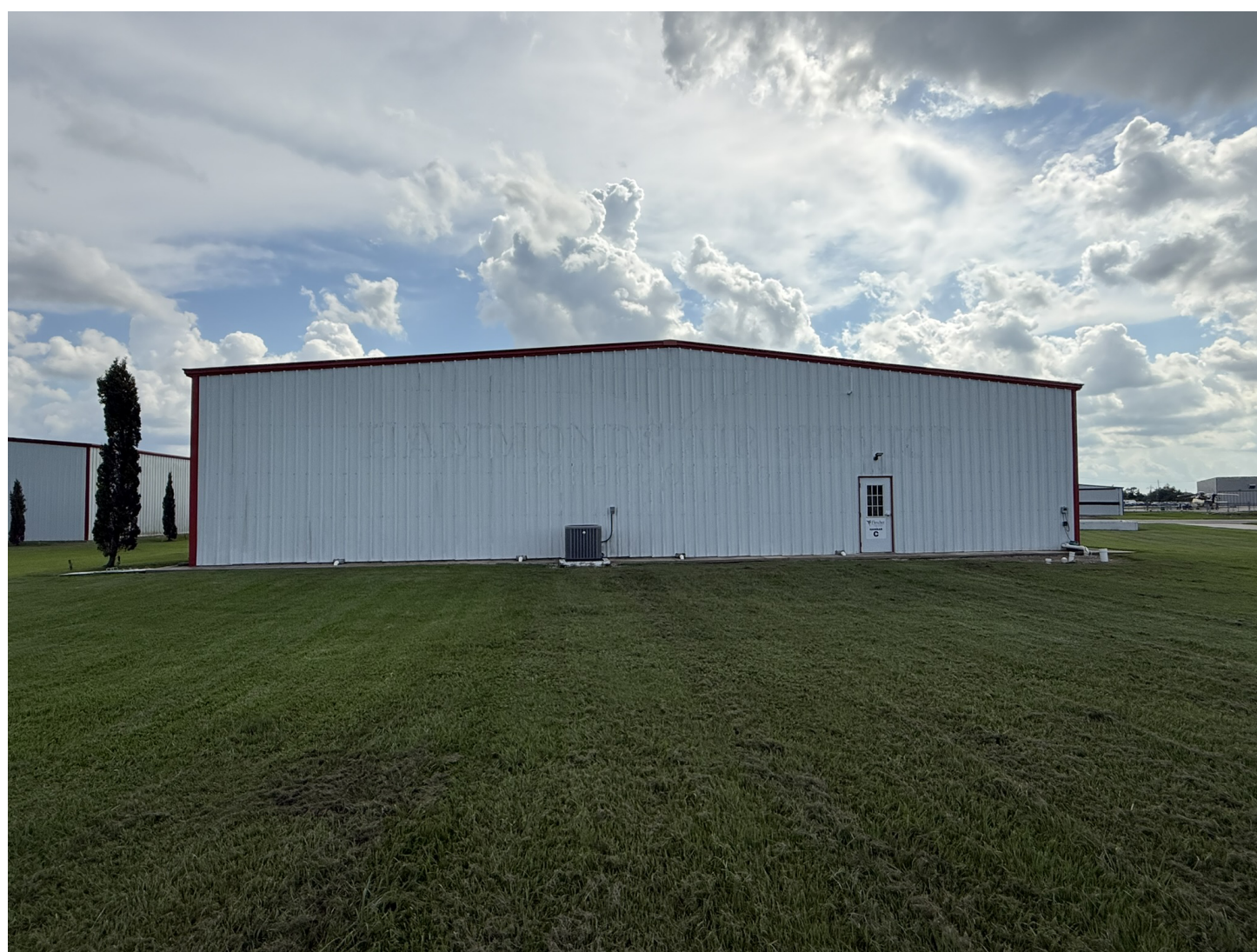
PHOTO OF WEST ELEVATION
