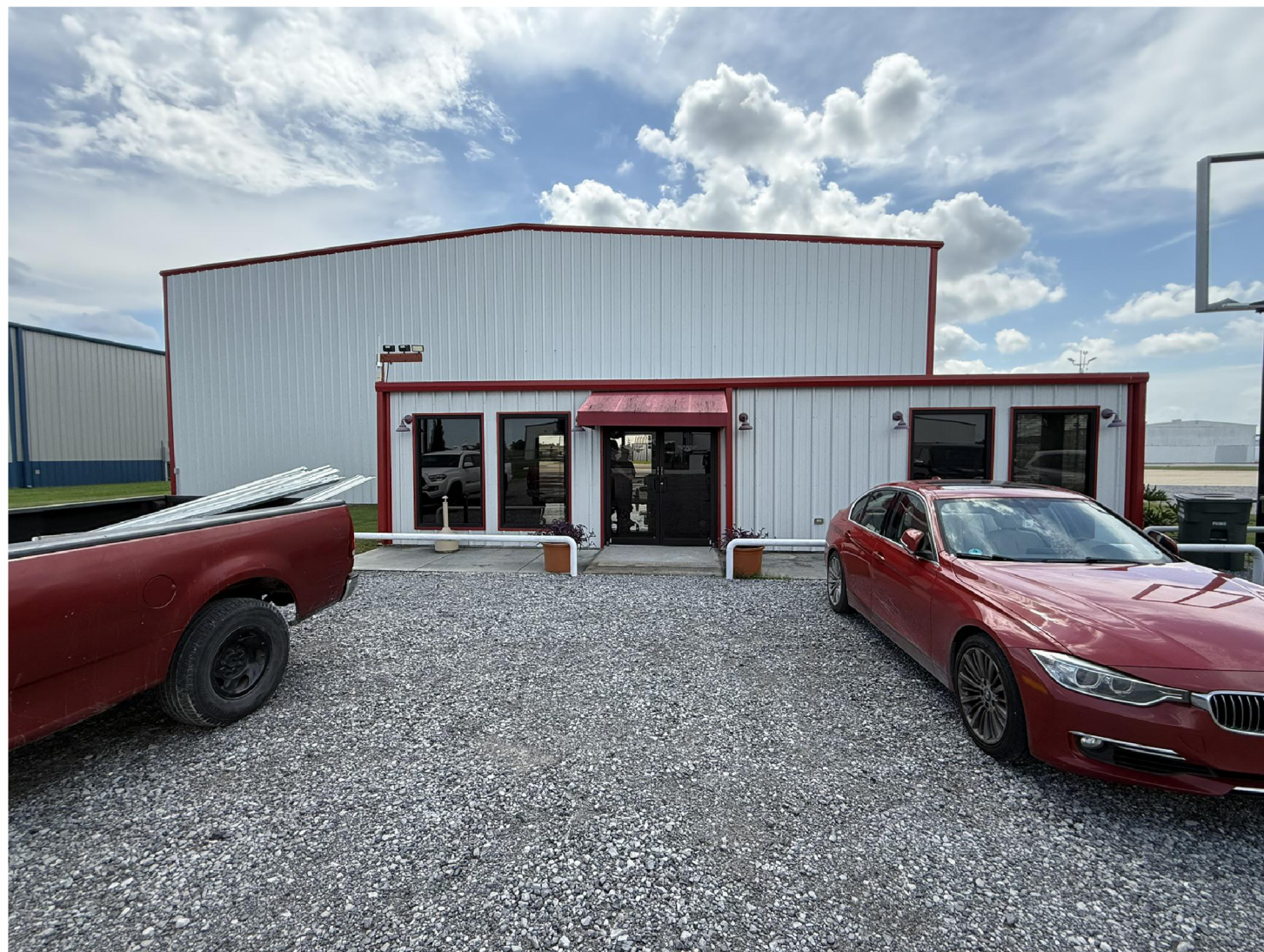
PHOTO OF EAST ELEVATION FOR REFERENCE
