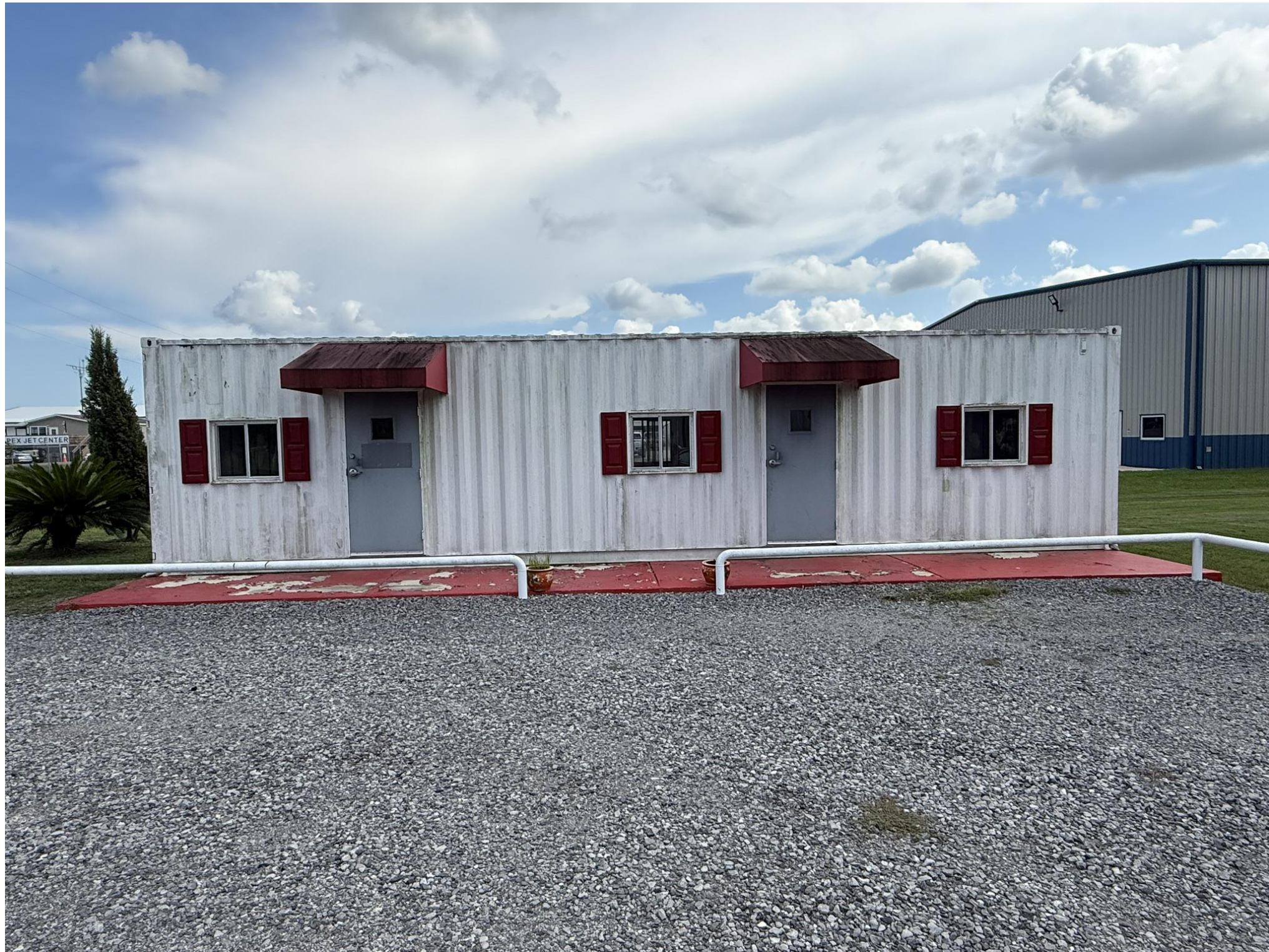
PRESSURE WASH BUILDING, REMOVE PLASTIC SHUTTERS, AND REPLACE CANOPY FABRIC WITH NEW FABRIC.
