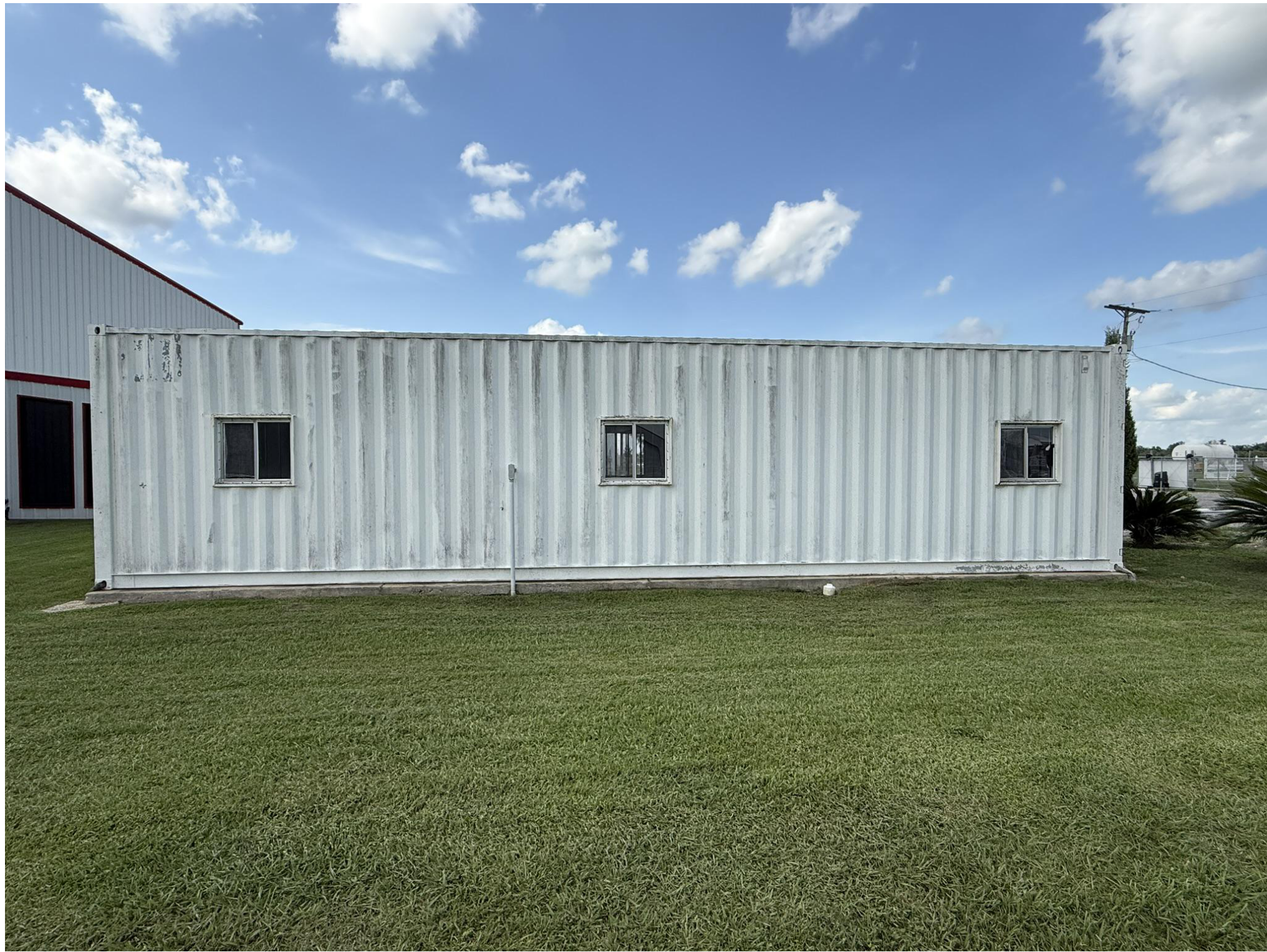
PRESSURE WASH BUILDING
