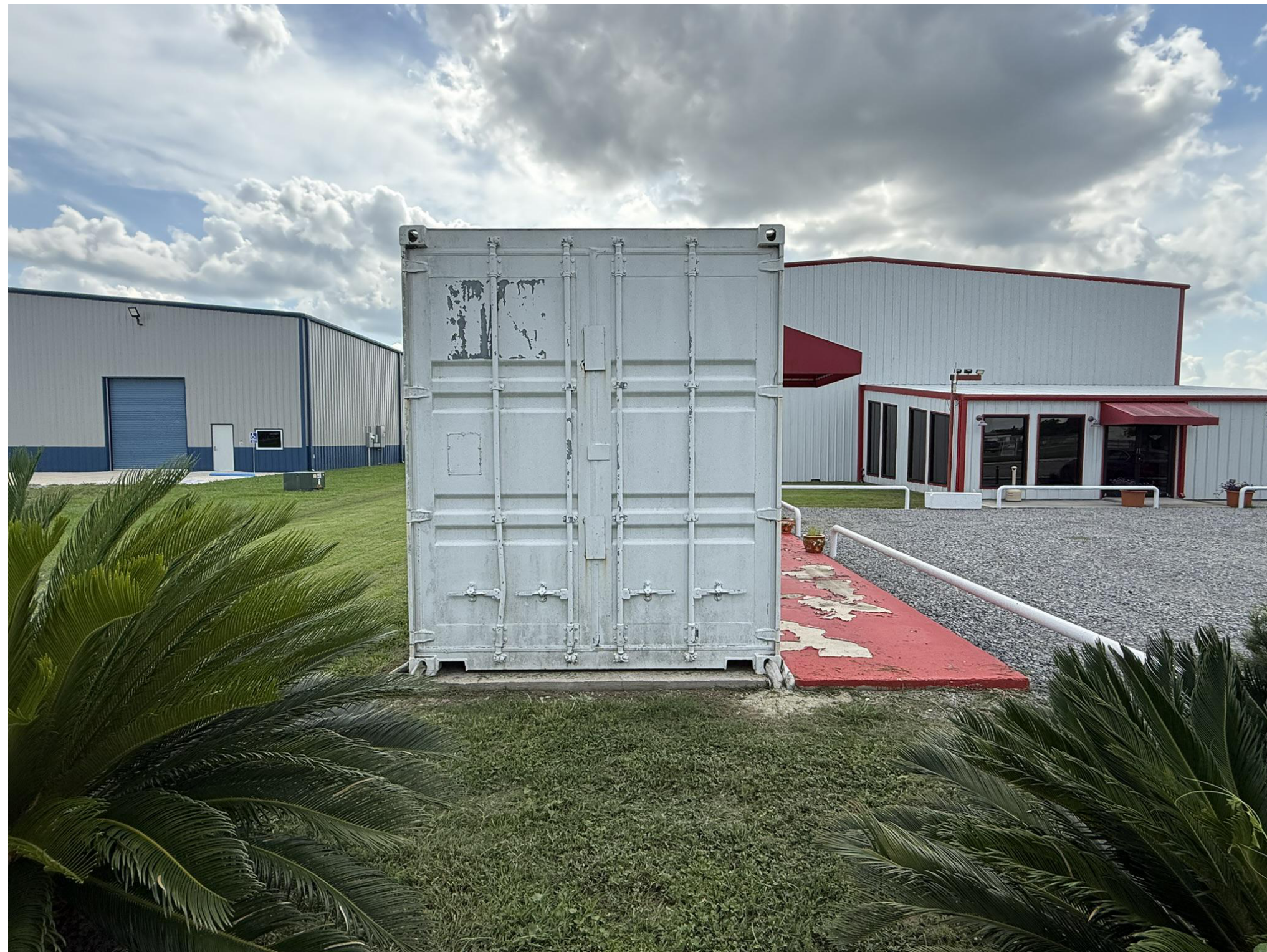
PRESSURE WASH BUILDING
