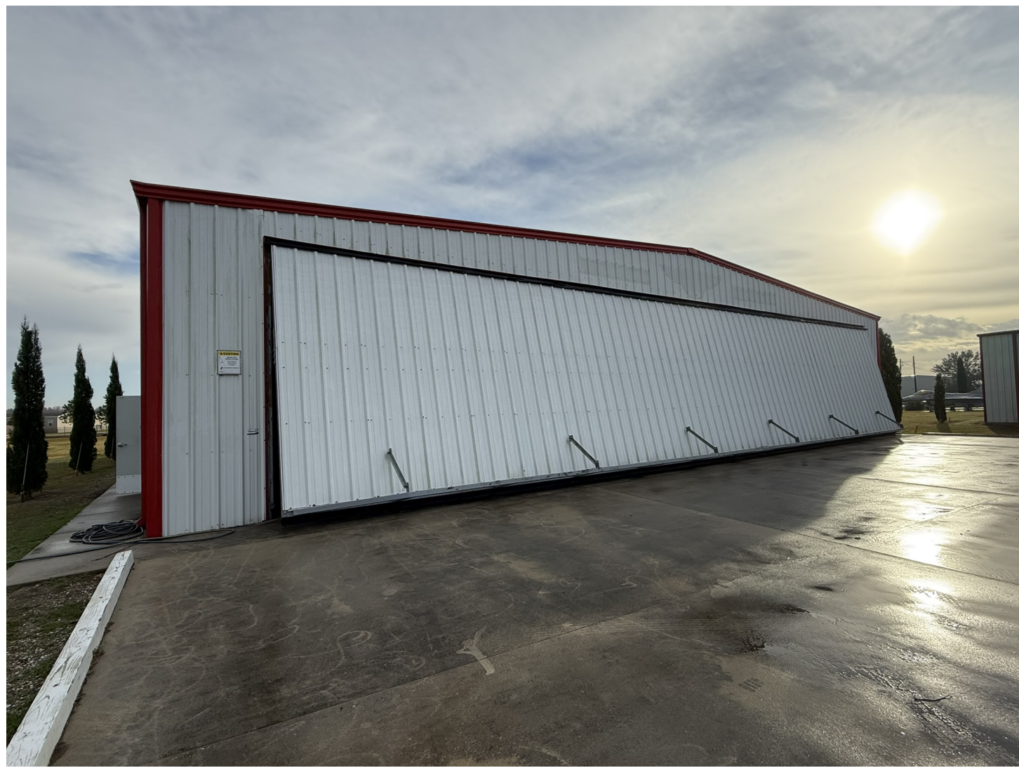
PHOTO OF WEST ELEVATION
