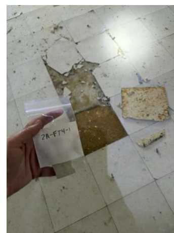
WHITE FLOOR TILE (2A-FT4-1, 1B-FT4-2)
