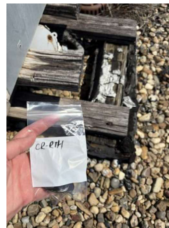
ROOFING TAR (CR-RT1-1, BR-RT1-2)
