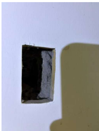
GREY WALL INSULATION (2C-WI1-1)
