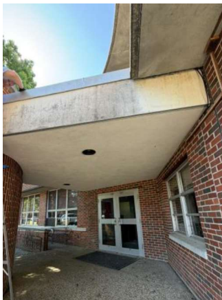
STUCCO COATING FRONT ENTRANCE (B1-SC1-1, B1-SC1-2, B1-SC1-3)
