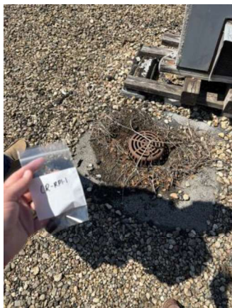
ROOF PATCH (CR-RP1-1)
