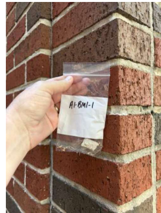
BRICK MORTAR (A1-BM1-1, C1-BM1-2, B1-BM1-3)
