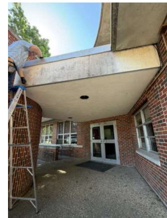
FLAT ROOF FRONT ENTRANCE (B1-FR1-1, B1-FR1-2)
