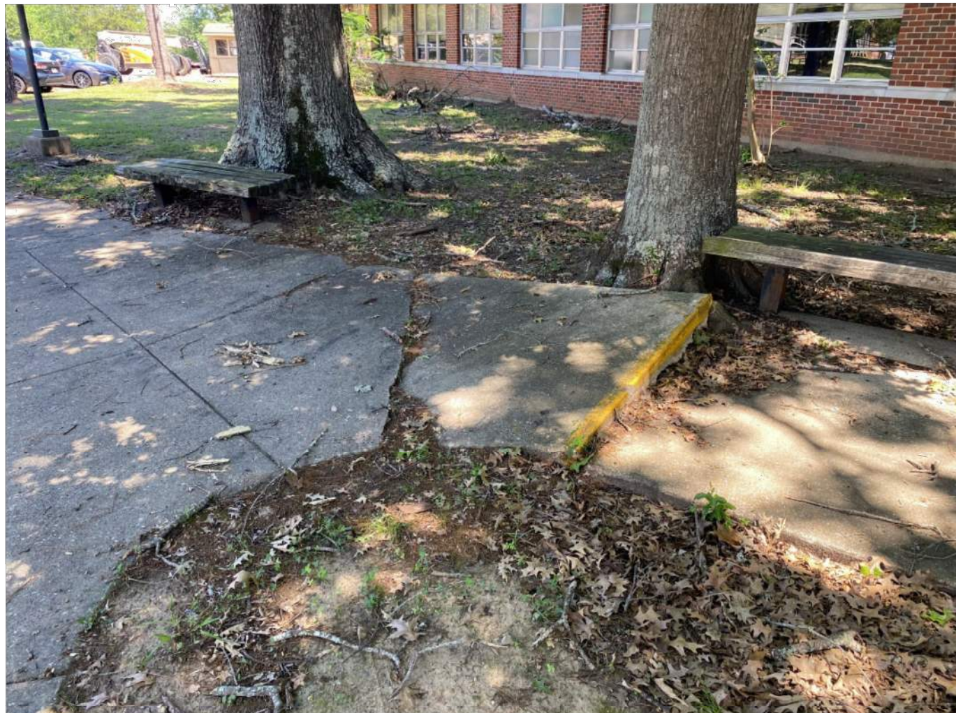
5/13/2026 TREES, SIDEWALK, BENCHES TO BE REMOVED IMG_0033.jpg
