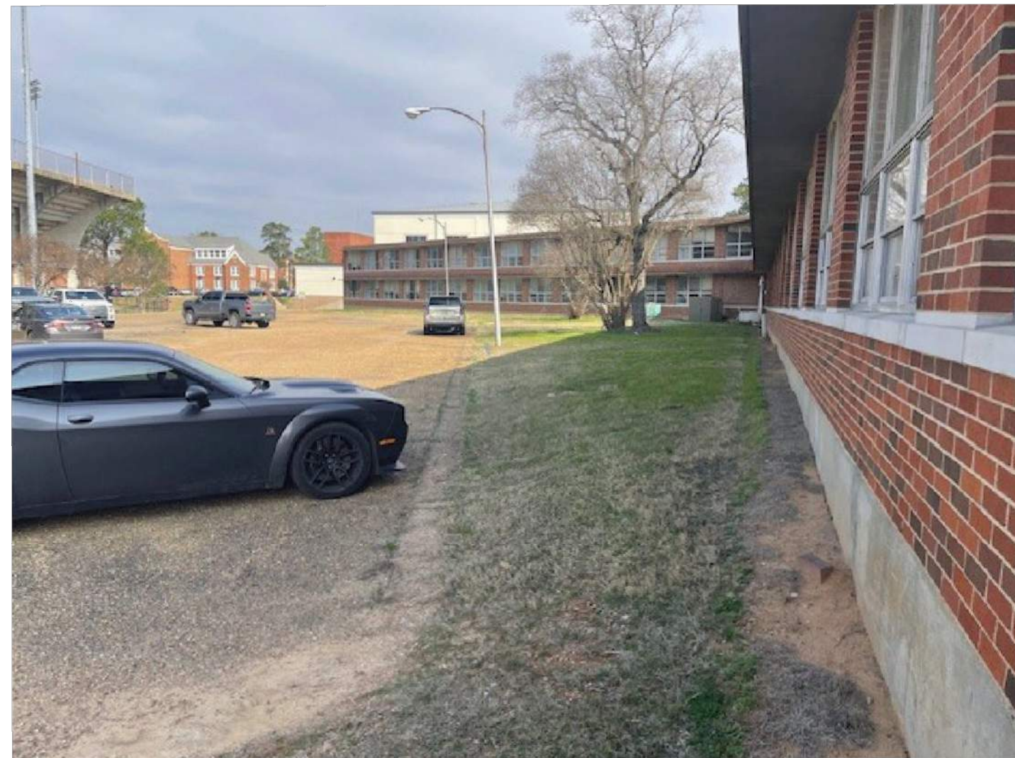
2/13/2026 SIGHT LIGHTING TO REMAIN Photo 27.jpg
