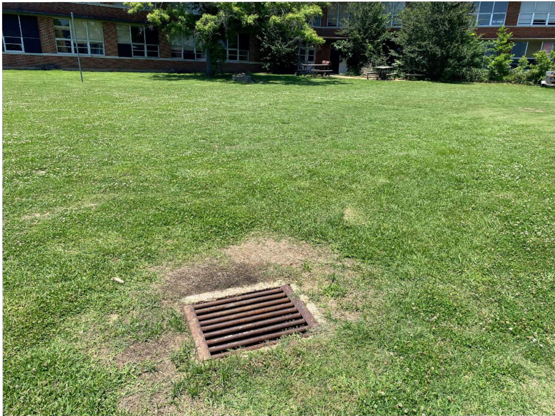
5/13/2026 STORM CATCH BASIN TO LEAVE & PROTECT IMG_9999.jpg
