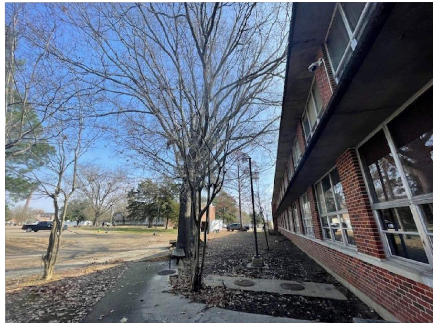
2/13/2026 LIGHTING, TREES, BENCHS TO BE REMOVED Photo 8.jpg
