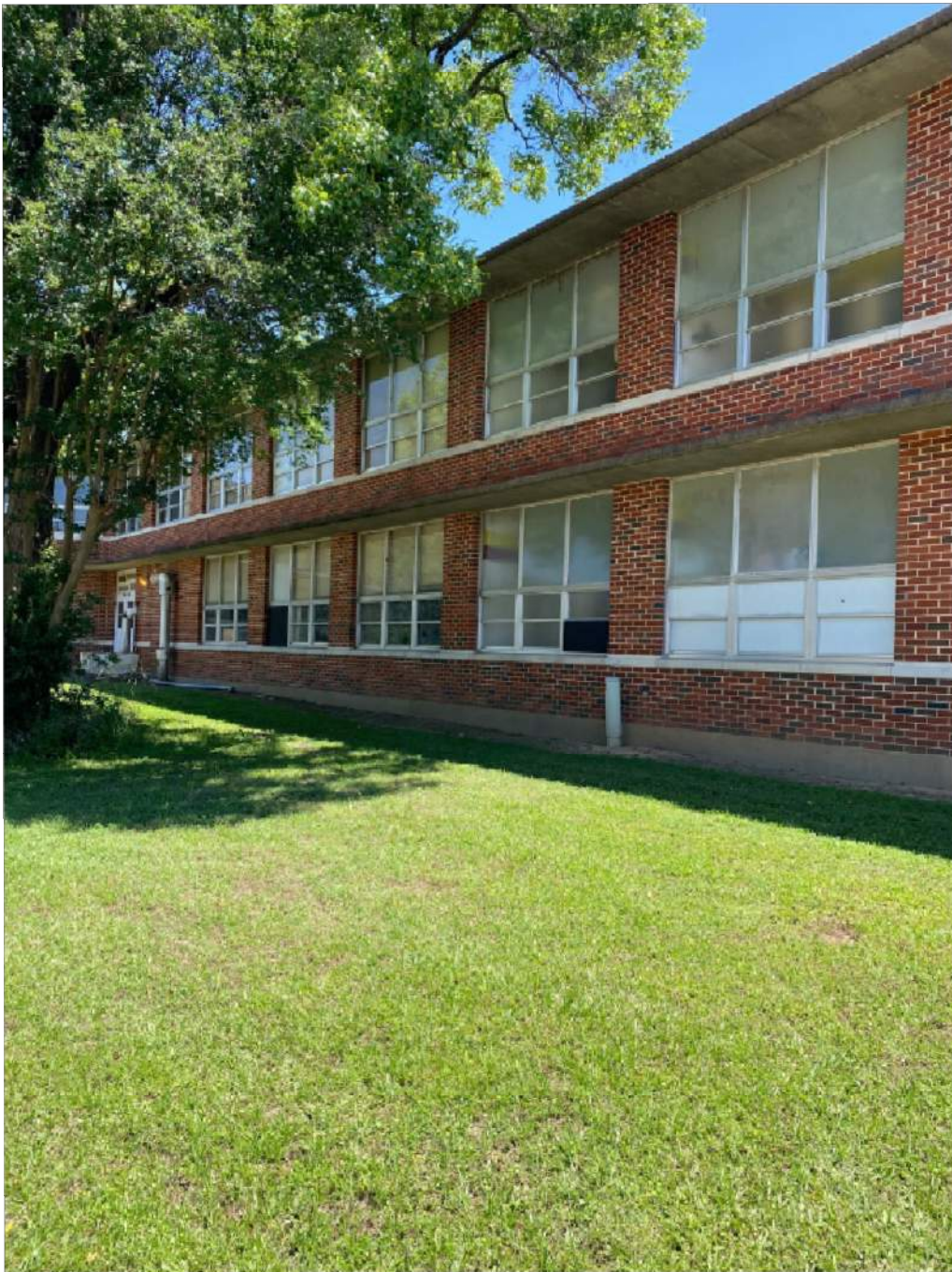
5/13/2026 TELECOM MARKER BY BUILDING TO REMOVE IMG_9980.jpg
