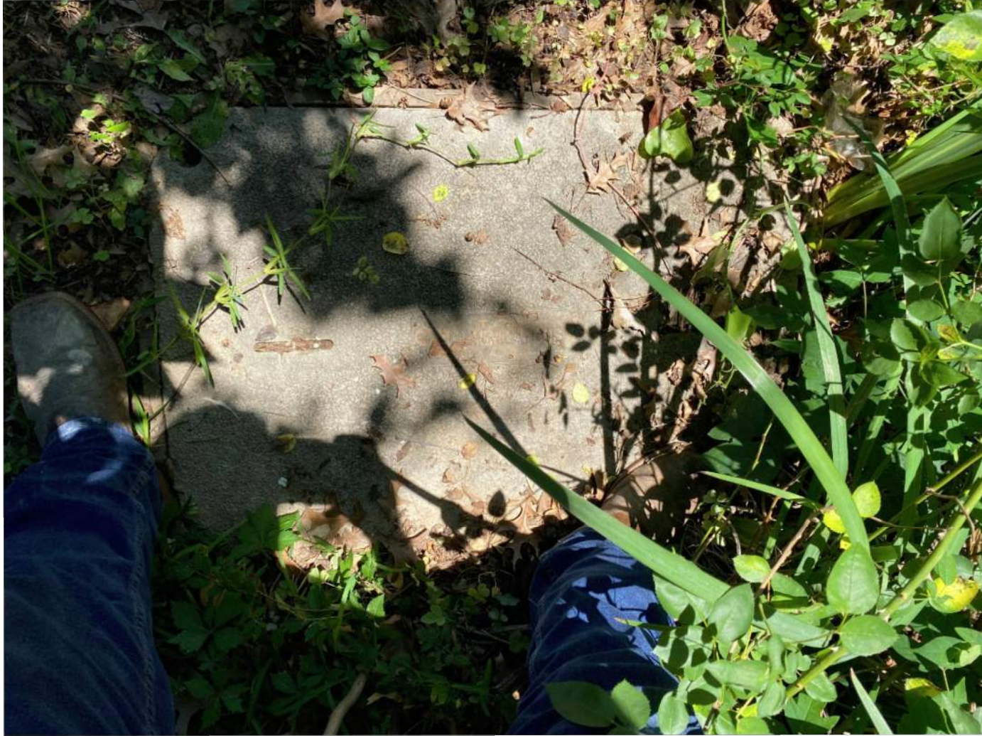
5/13/2026 EXISTING TELECOM CABINET AND UNDERGROUND FIBER OPTIC UTILITIES SHALL REMAIN IN SERVICE. PROTECT THROUGHOUT CONSTRUCTION.IMG_9988.jpg
