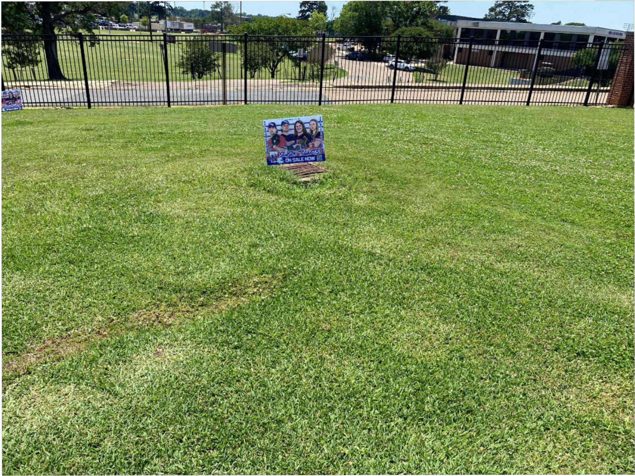
5/13/2026 STORM CATCH BASIN TO LEAVE & PROTECT IMG_0006.jpg
