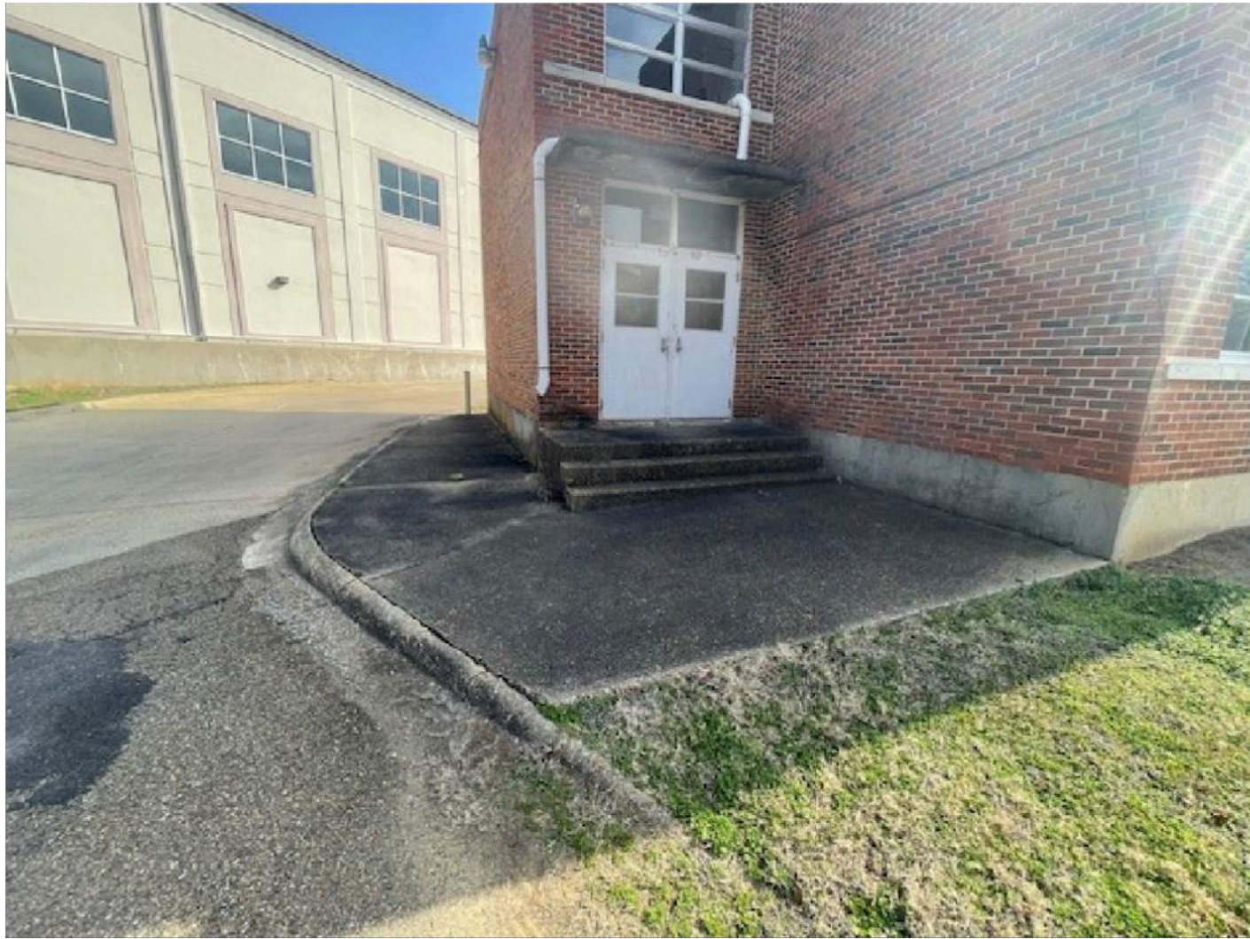
2/13/2026 SIDEWALK PAVING TO BE REMOVED TO CURB Photo 1.jpg
