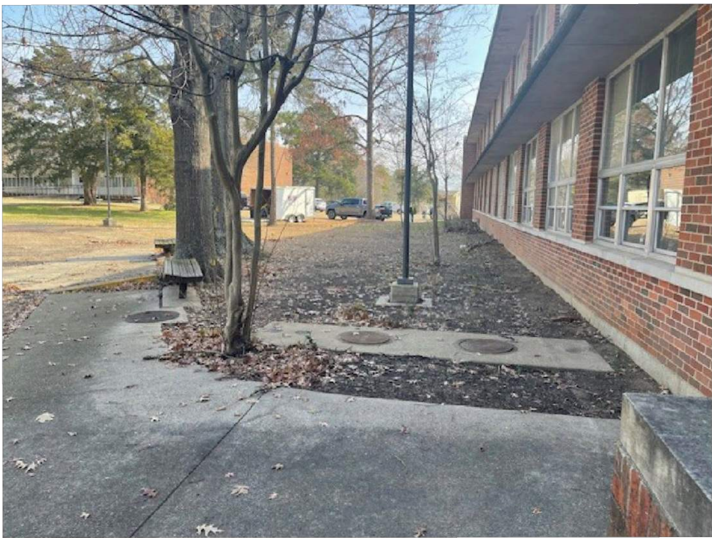
2/13/2026 MANHOLE TO REMAIN Photo 7.jpg
