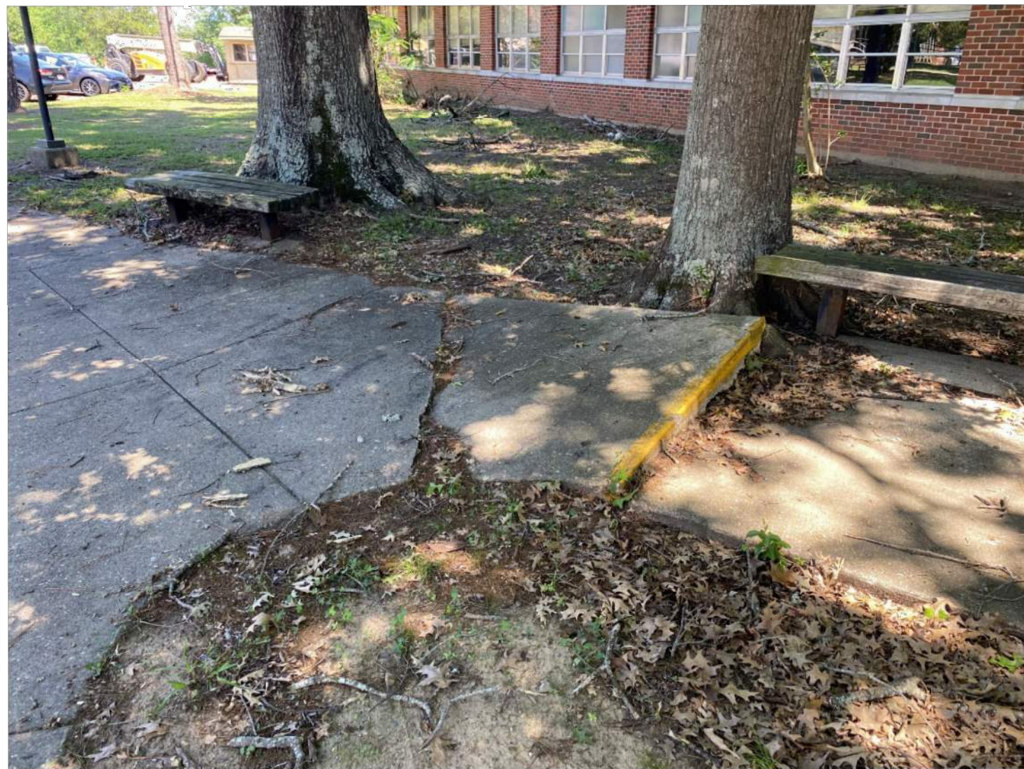
5/13/2026 TREES, SIDEWALK, BENCHES TO BE REMOVED IMG_0033.jpg
