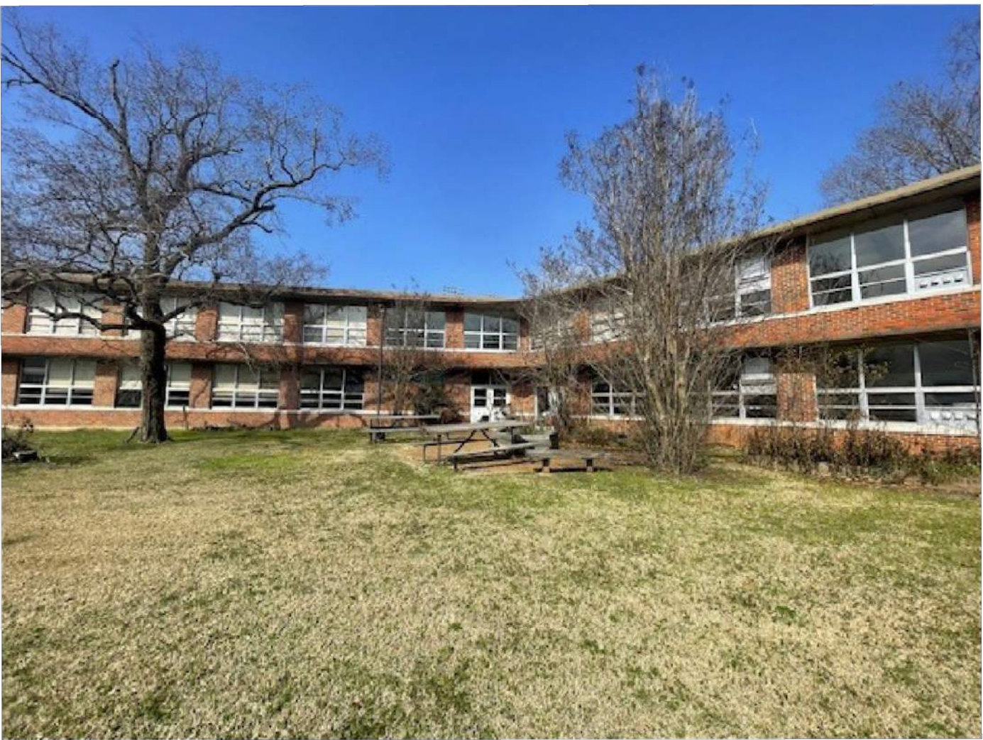
2/13/2026 TREES, PLANTERS, SIDEWALK TO BE REMOVED Photo 19.jpg
