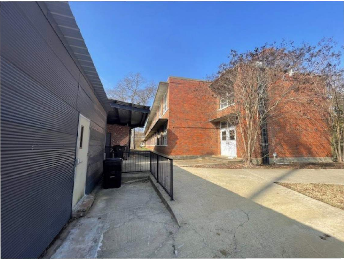
2/13/2026 HVAC LINES TO BE CUT & CAPPED @ BLDG Photo 15.jpg
