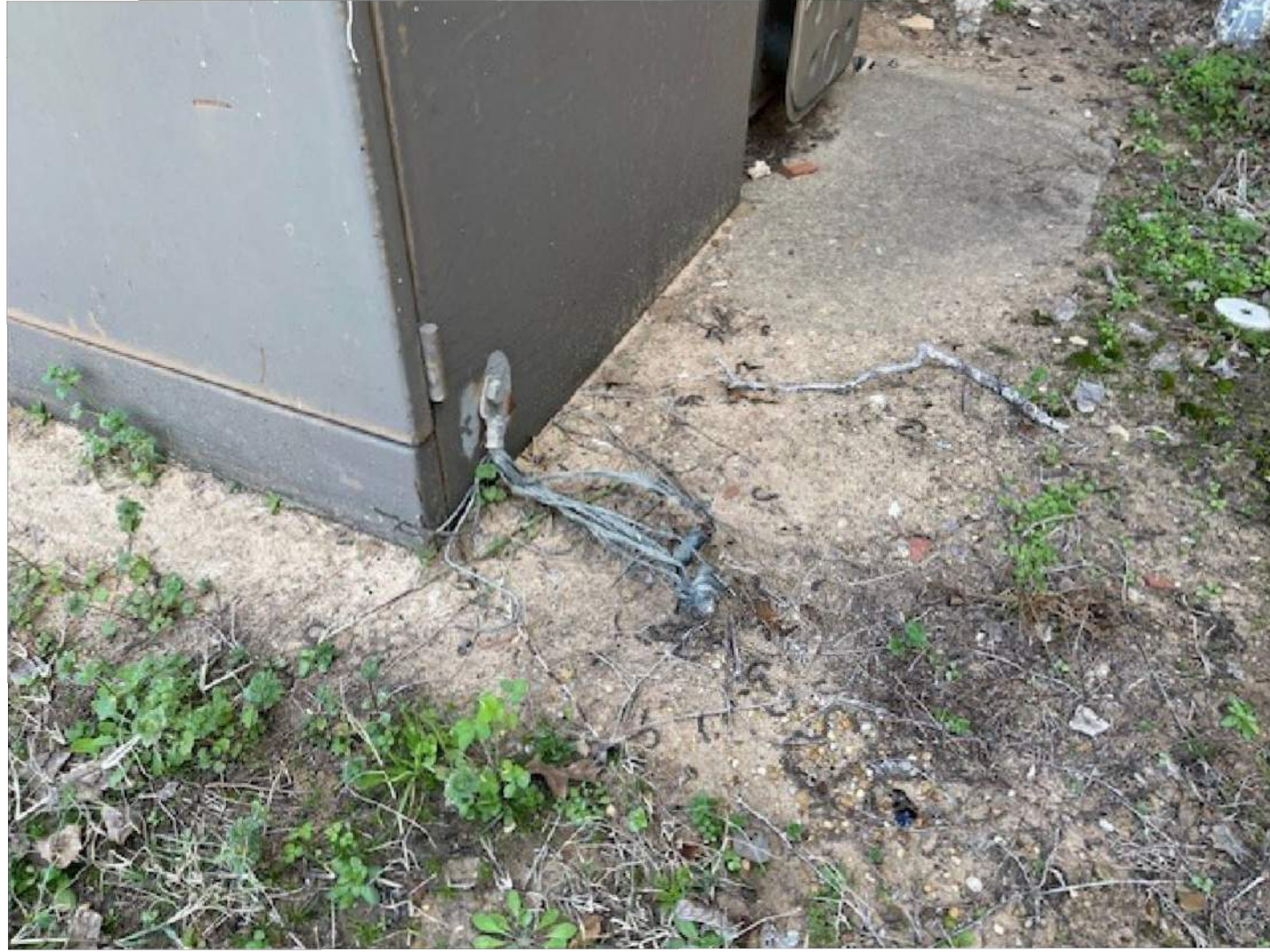
2/13/2026 REPAIR GROUND WIRE Photo 32.jpg
