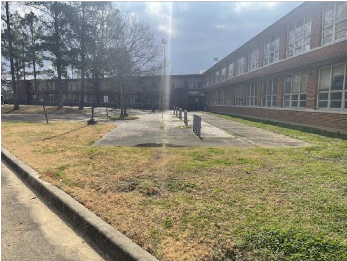
2/13/2026 SIDEWALK & BIKE RACKS TO BE REMOVED Photo 3.jpg
