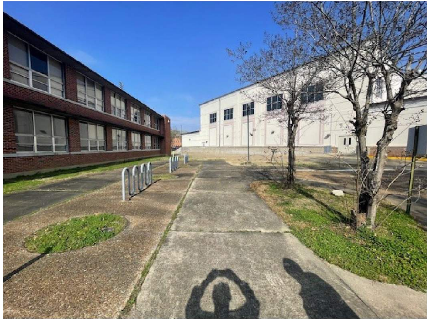
2/13/2026 REMOVE SIDEWALKS, SITE PAVING, AND BIKE RACKS. Photo 4.jpg
