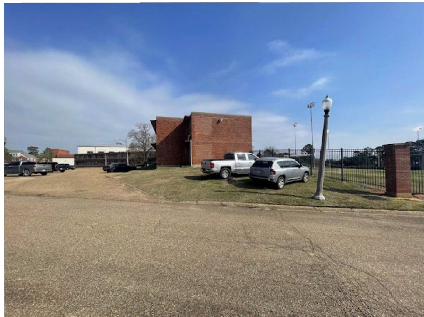
2/13/2026 SITE LIGHTING TO REMAIN Photo 24.jpg
