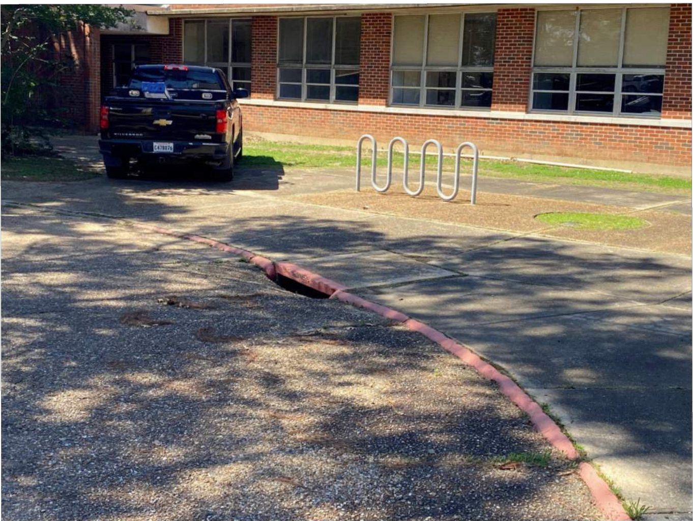
5/13/2026 ENTRY DRIVEWAY STORM CATCH BASIN TO PROTECT IMG_9974.jpg
