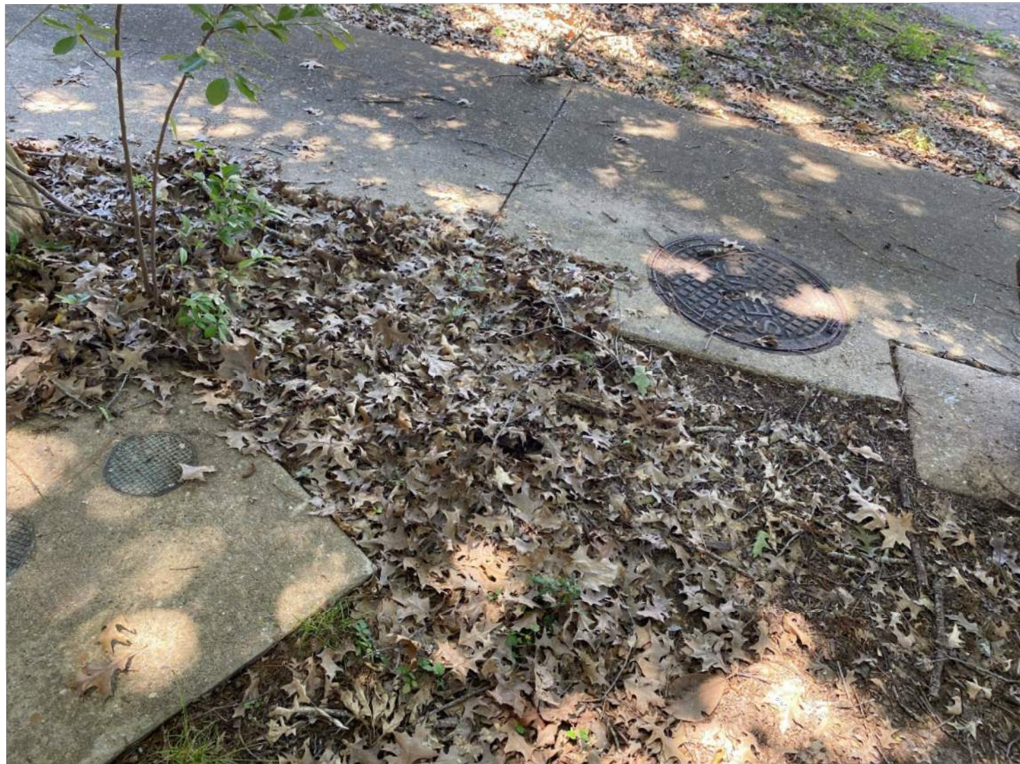
5/13/2026 SEWER MANHOLE TO REMAIN & PROTECT IMG_0016.jpg
