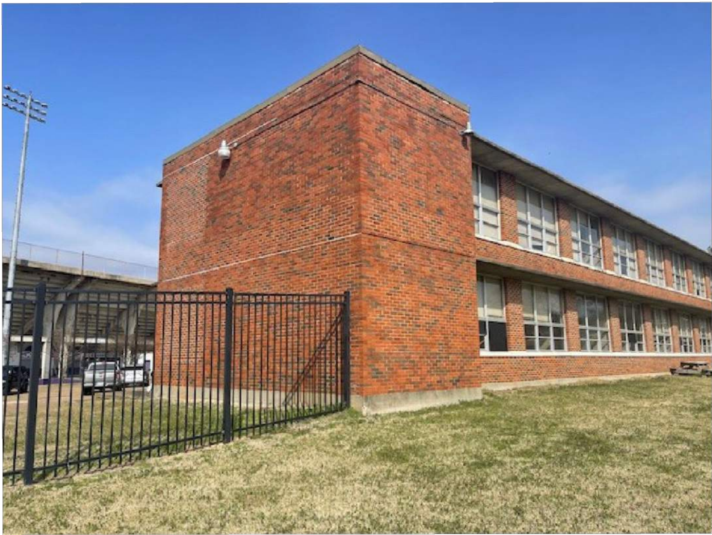
2/13/2026 PORTION OF FENCE REMOVED BY BLDG Photo 21.jpg
