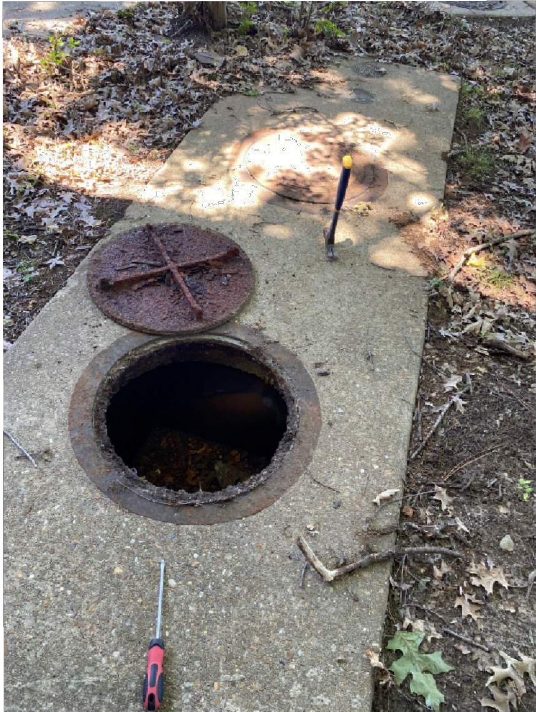
5/13/2026 CONCRETE MANHOLE BOX TO REMOVE. VERIFY THE CONTENTS OF THE MANHOLE PRIOR TO DEMOLITION TO DETERMINE WHETHER IT IS ACTIVE OR ABANDONED SERVICE. IMG_0013.jpg
