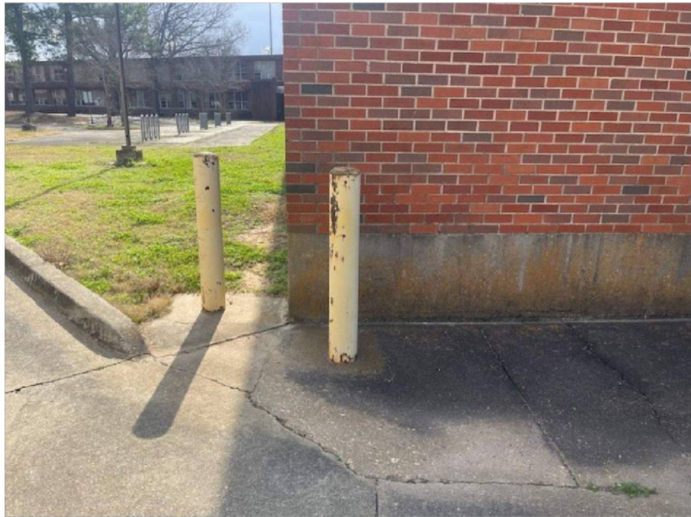
2/13/2026 SAWCUT SIDEWALK PAVING DRIVE TO REMAIN Photo 2.jpg
