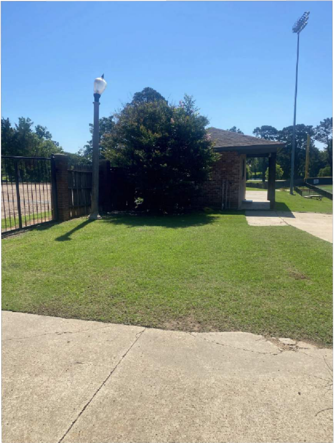
5/13/2026 LOCATION TO CUT/CAP HWS/R PIPES IMG_9951.jpg
