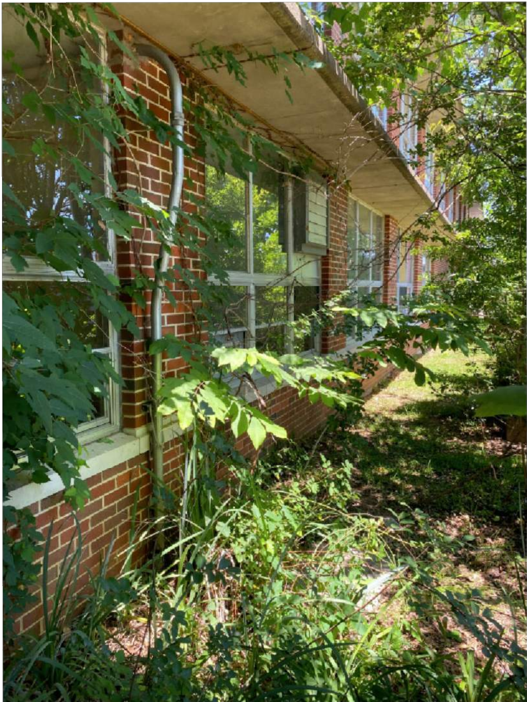
5/13/2026 TELECOM BOX CONDUIT ENTERS BLDG TO REMOVE IMG_9989.jpg
