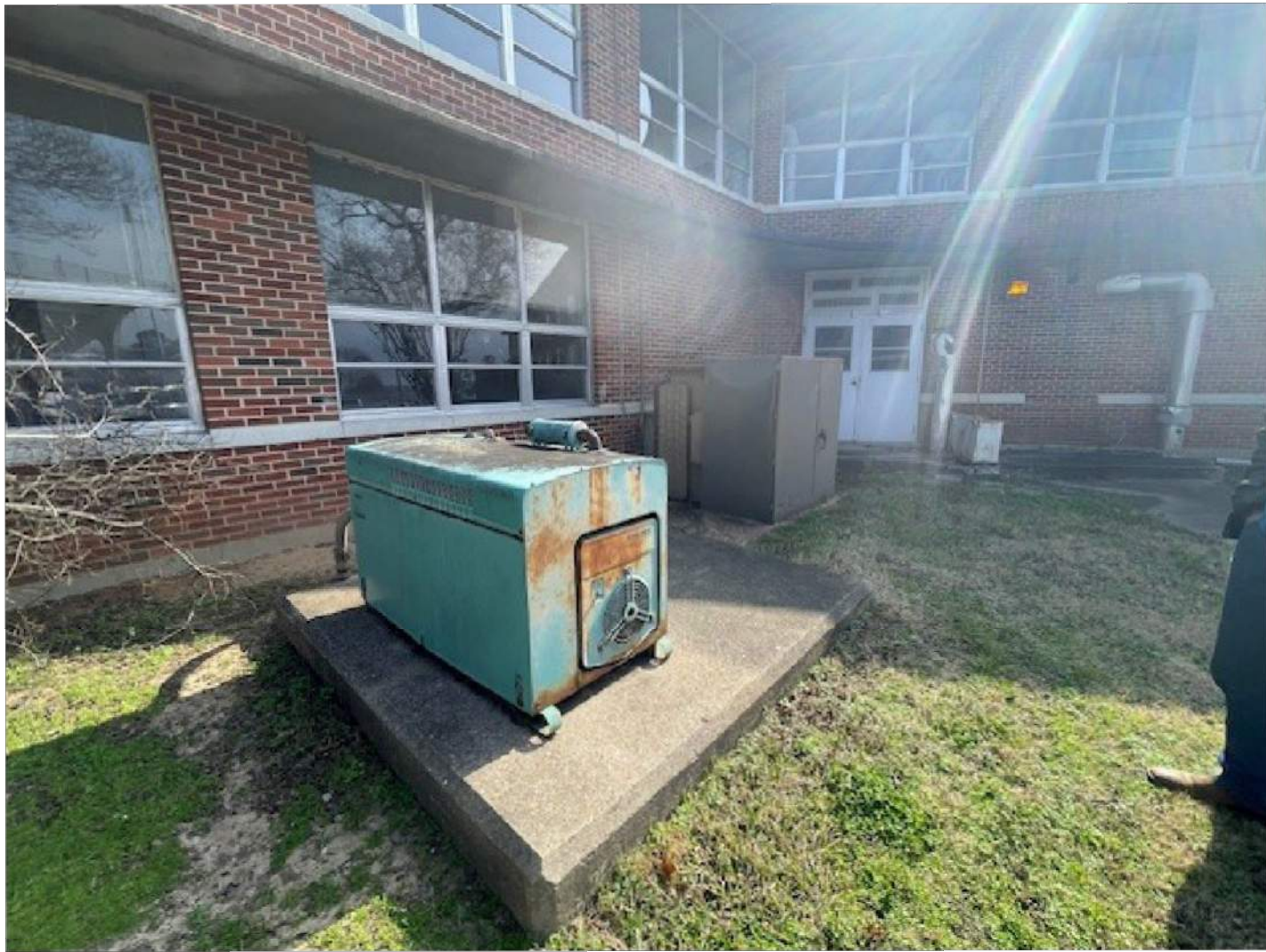
2/13/2026 GENERATOR & PAD TO BE REMOVED Photo 29.jpg
