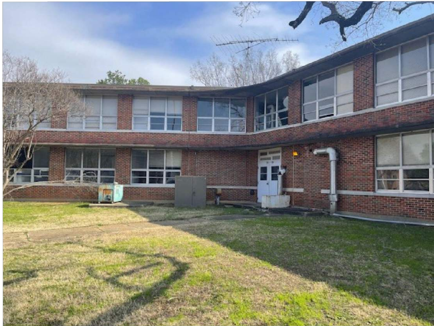
2/13/2026 SIDEWALK TO BE REMOVED Photo 28.jpg
