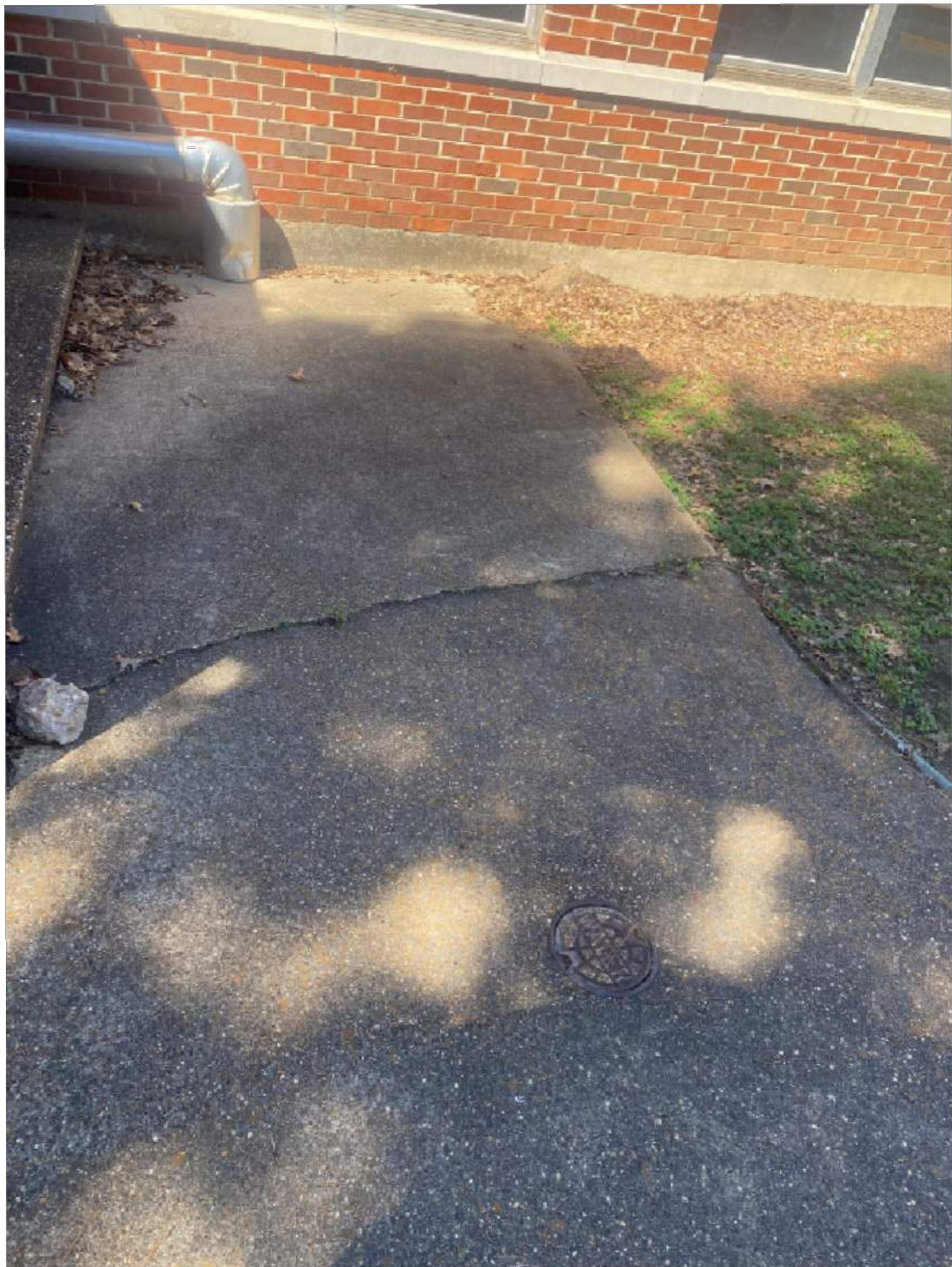
5/13/2026 WATER VALVE @ MAIN ENTRY SIDEWALK IMG_9948.jpg
