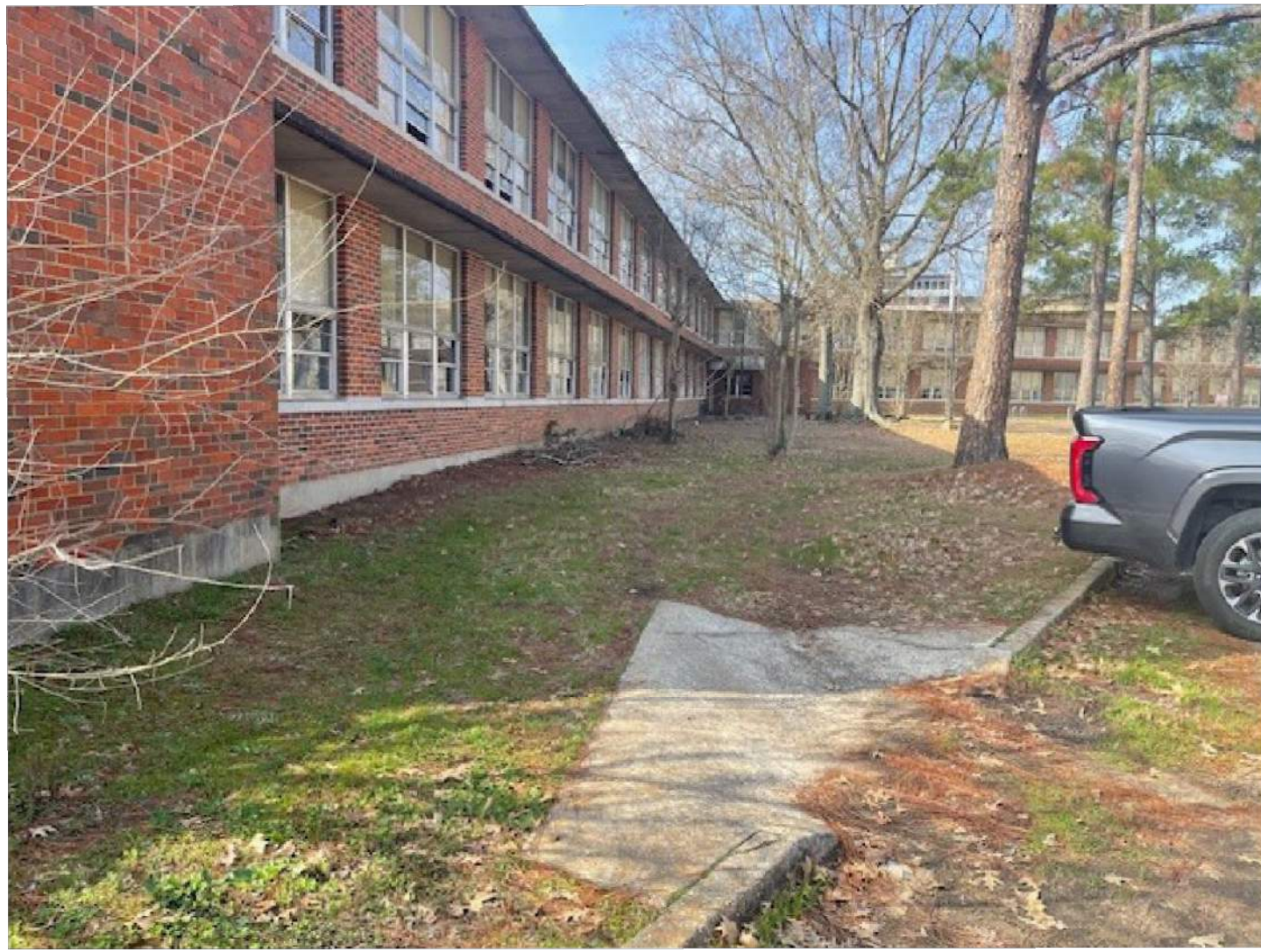
2/13/2026 BUILDING & TREES TO BE REMOVED Photo 13.jpg
