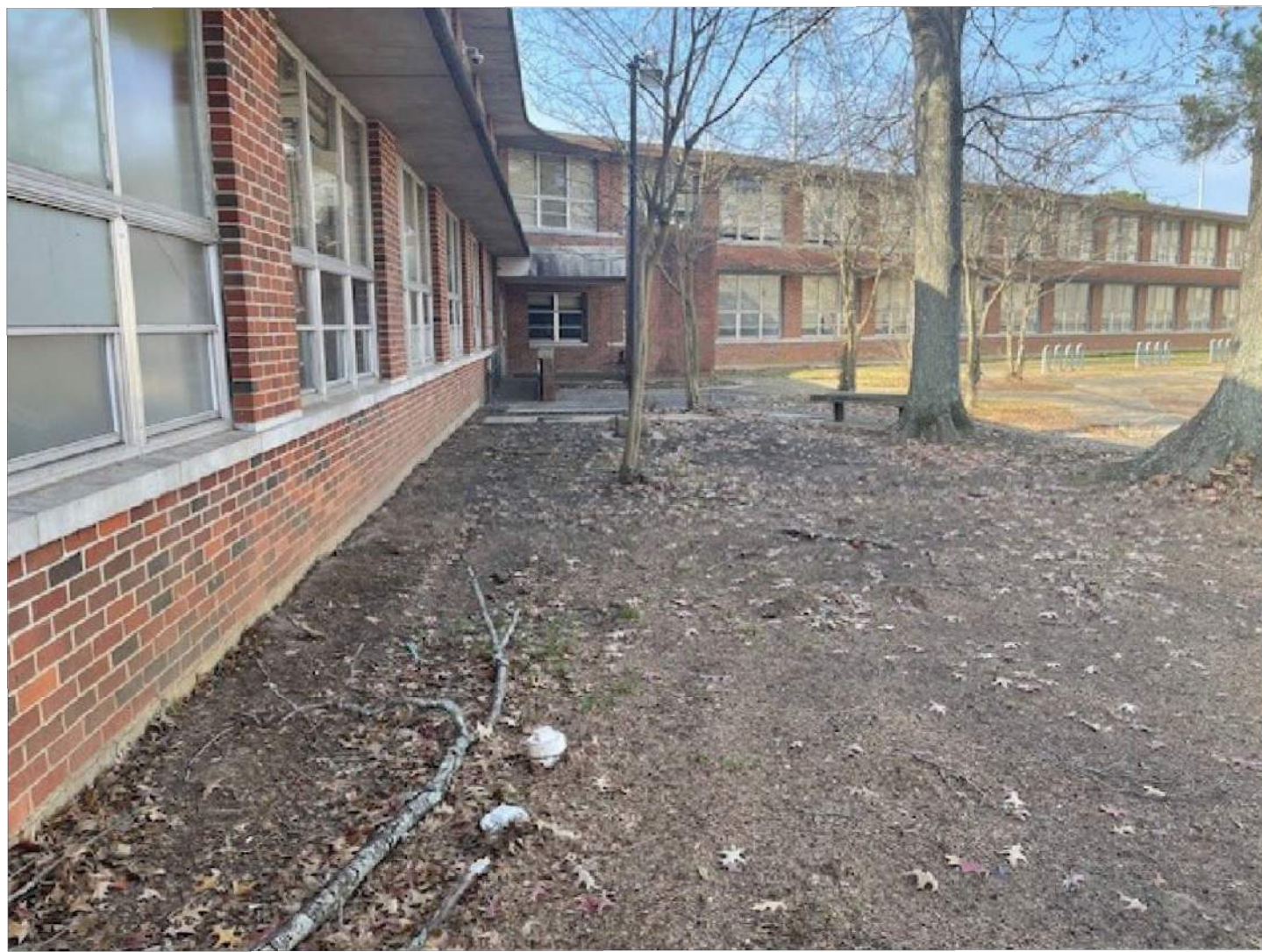
2/13/2026 SANITARY SEWER TO BE REMOVED TO MANHOLE Photo 12.jpg
