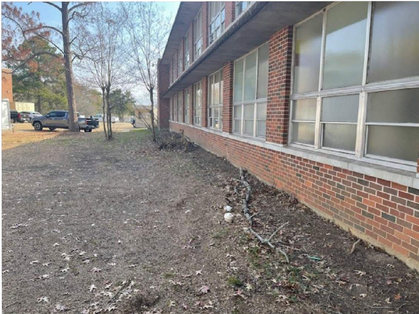
2/13/2026 SANITARY SEWER TO BE REMOVED TO MANHOLE Photo 11.jpg
