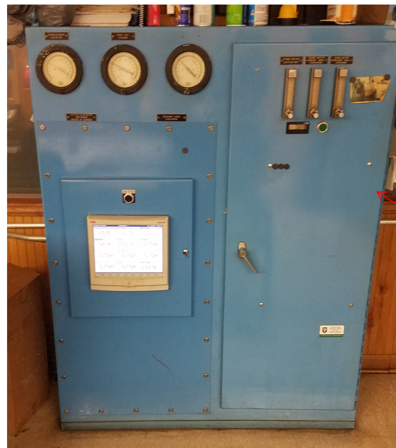
Existing PLC Cabinet - PLC rack located on interior of door.
