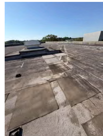
LEVEL 3 ROOF VIEW
