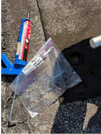
MG-11 ROOF CORE SAMPLE
