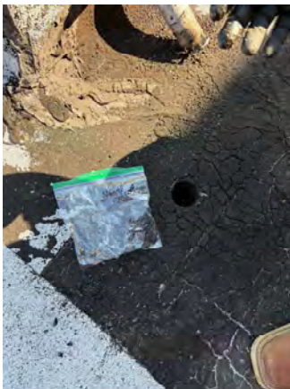
MG-6 ROOF CORE SAMPLE
