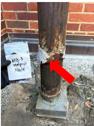
MG-3 VENT PIPE SILVER PAINT & BLACK CAULK
