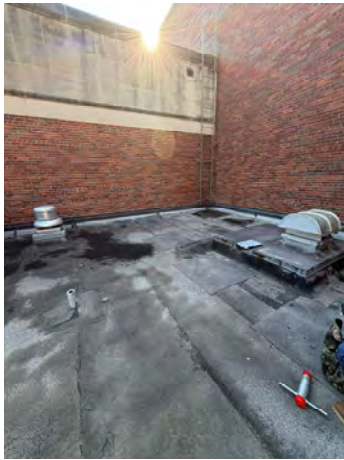
LEVEL 1 ROOF VIEW NW SIDE
