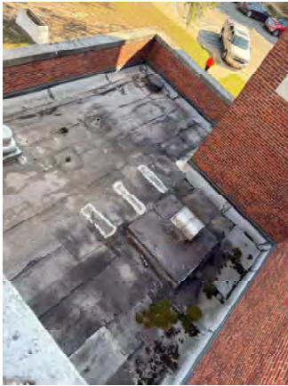
LEVEL 1 ROOF VIEW NE SIDE
