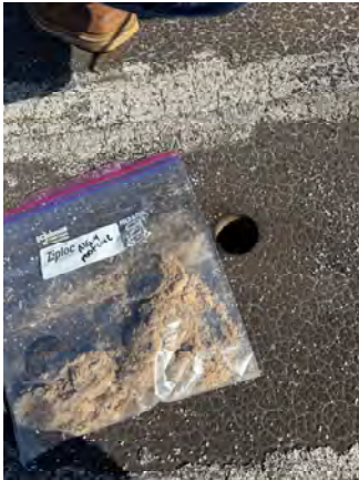
MG-9 ROOF CORE SAMPLE
