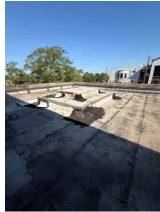
LEVEL 2 ROOF VIEW
