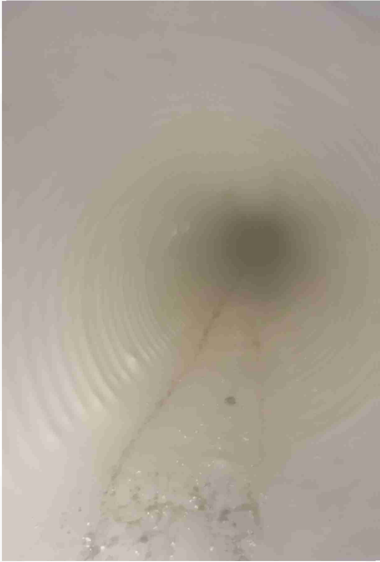
After Thermoform PVC Lining
