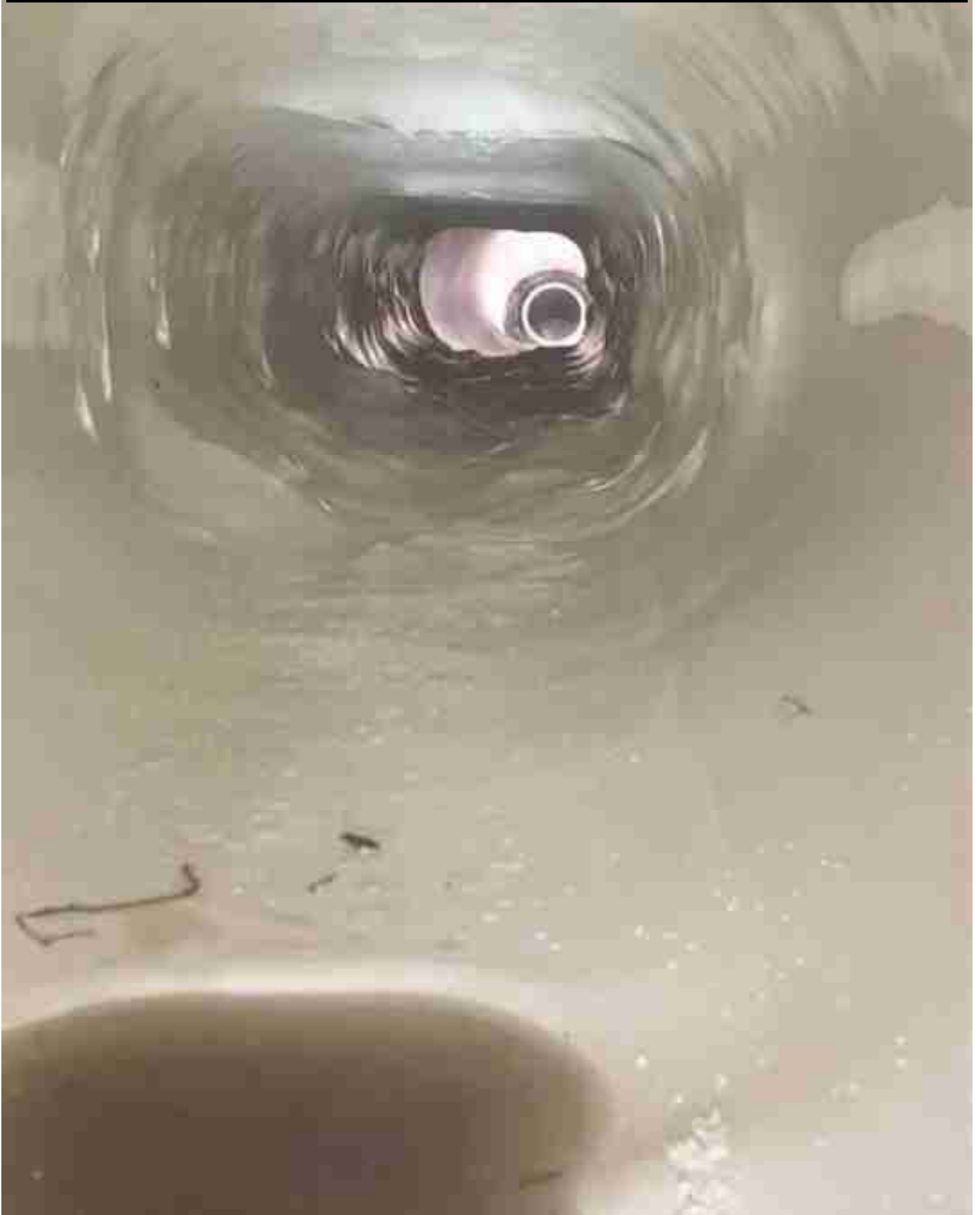
Stone laid culvert lined with Thermoform PVC Lining showing the versatility of Thermoform.
