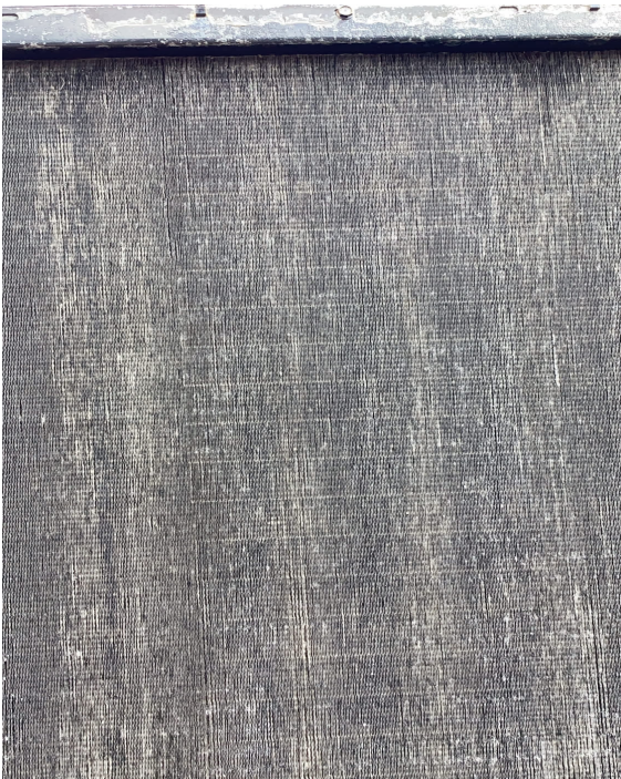
Chiller coils after cleaning
