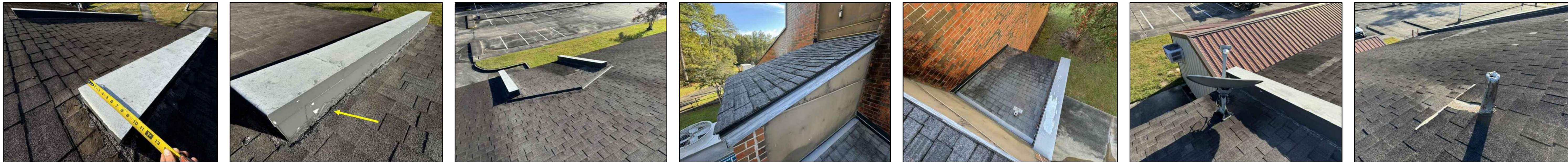
EXISTING CONDITION PHOTOS
