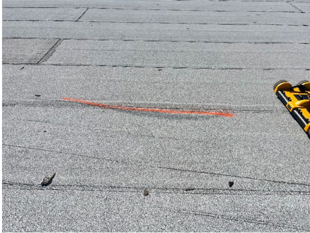
Blisters in the cap sheet membrane
