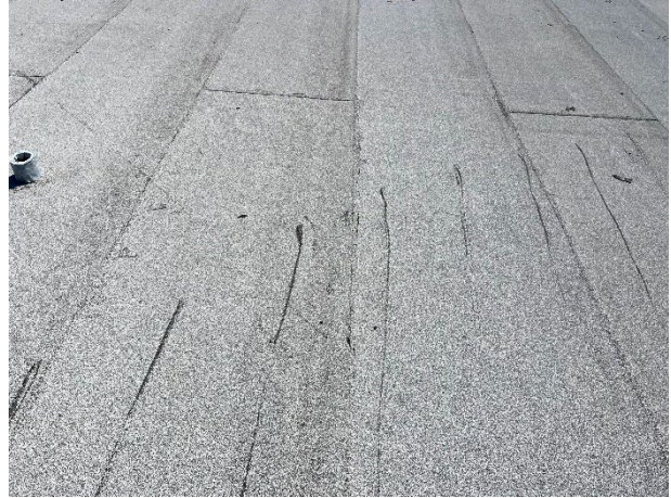
Damaged cap sheet membrane observed at numerous locations
