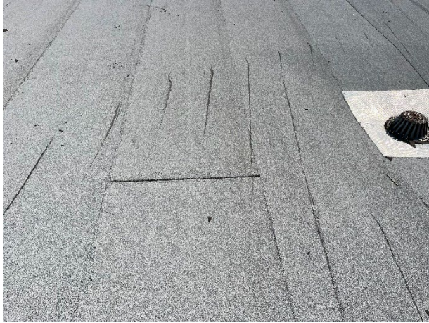
Damaged cap sheet membrane observed at numerous locations
