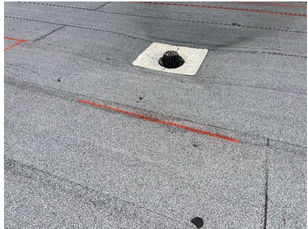
Blisters in the cap sheet membrane
