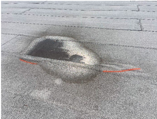
Blisters in the cap sheet membrane
