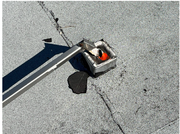
Damaged pitch pans for the mechanical equipment tie down straps
