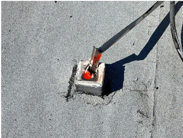
Damaged pitch pans for the mechanical equipment tie down straps
