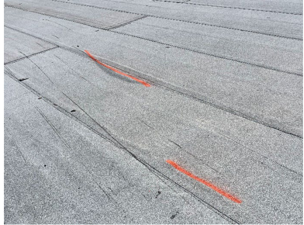
Blisters in the cap sheet membrane
