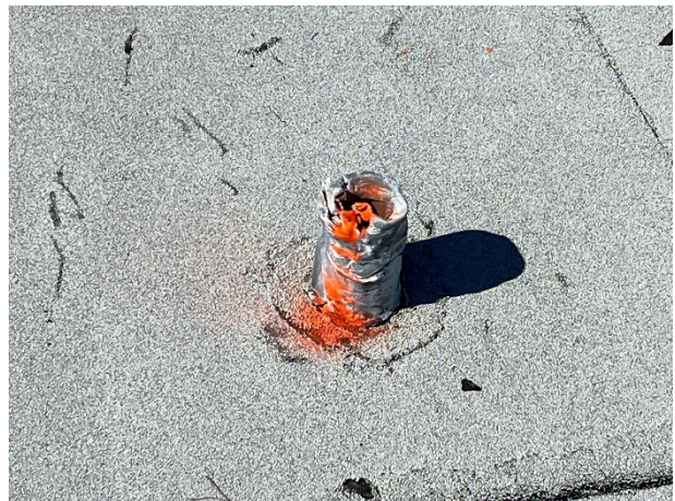
Damaged lead roof jacks
