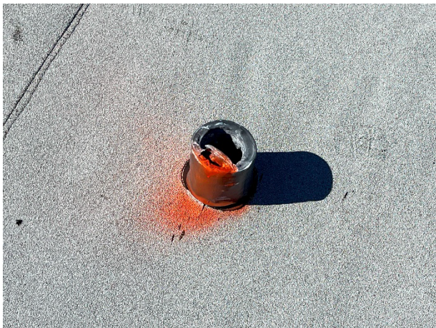
Damaged lead roof jacks
