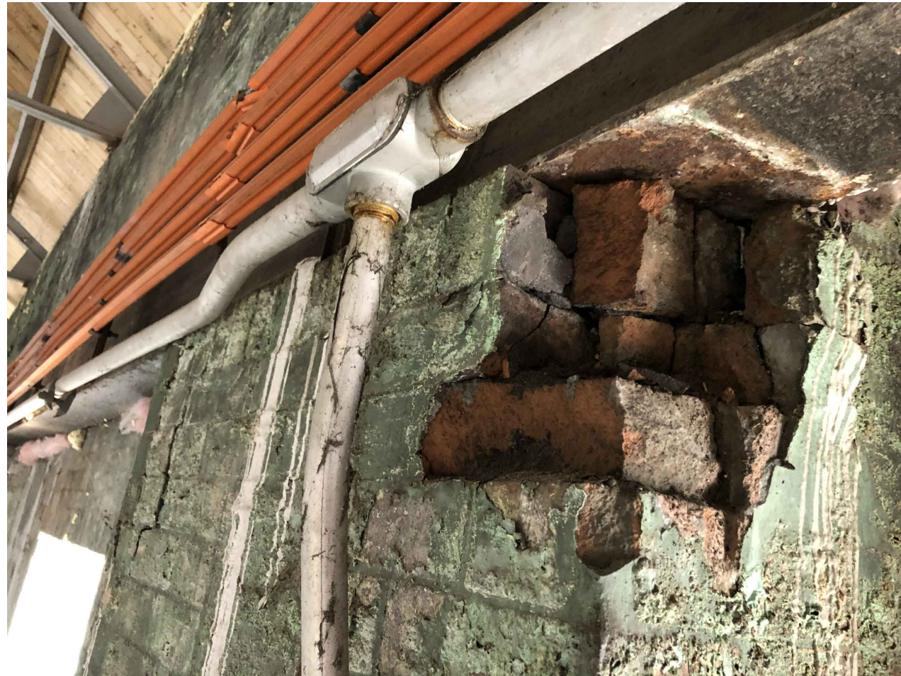
SAMPLE OF ITEM: (L) BRICK PILASTER SUPPORT FAILURE
