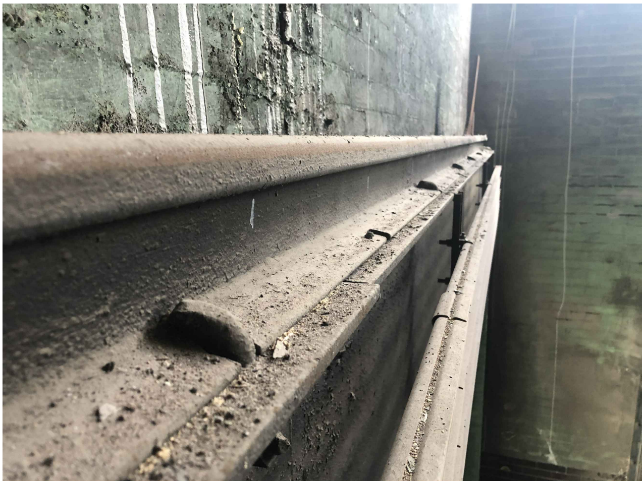
SAMPLE OF ITEM: (B) RAIL TO RUNWAY BEAM ANCHOR MISSING
