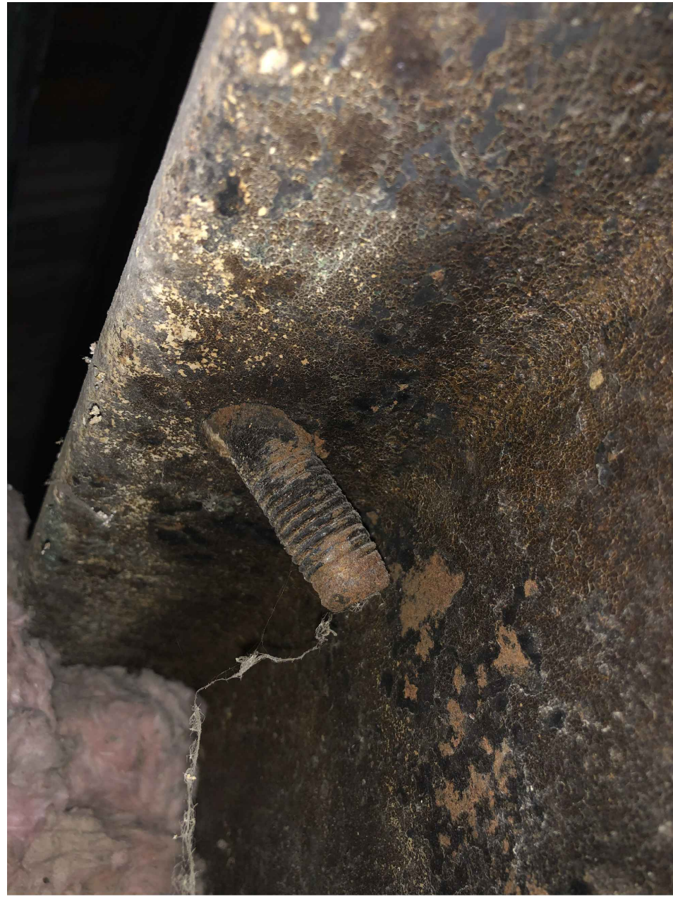
SAMPLE OF ITEM: (B) RAIL TO RUNWAY BEAM ANCHOR MISSING NUT
