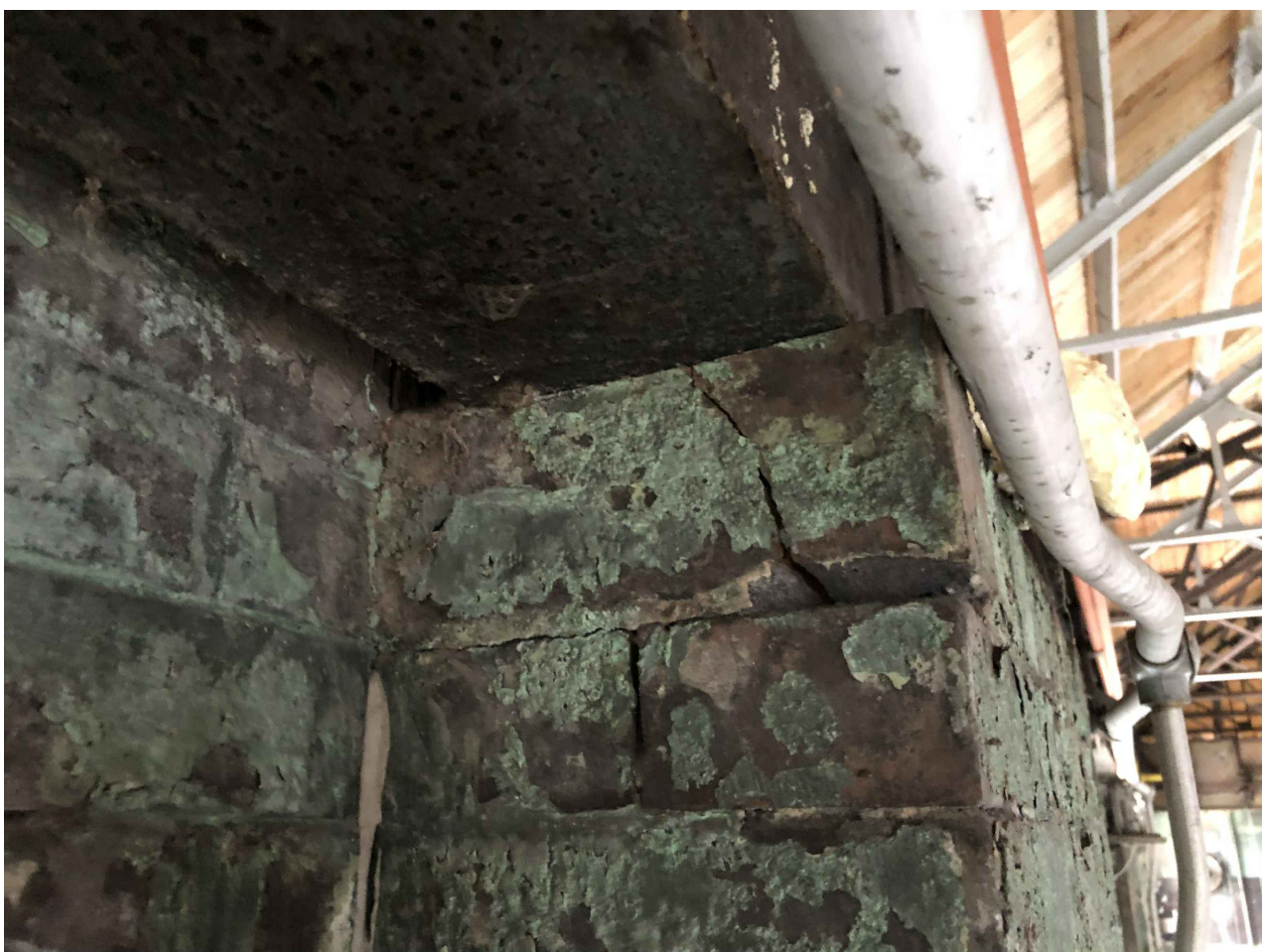
SAMPLE OF ITEM: (J) PILASTER BRICK CRACKS AND MORTAR FAILURE
