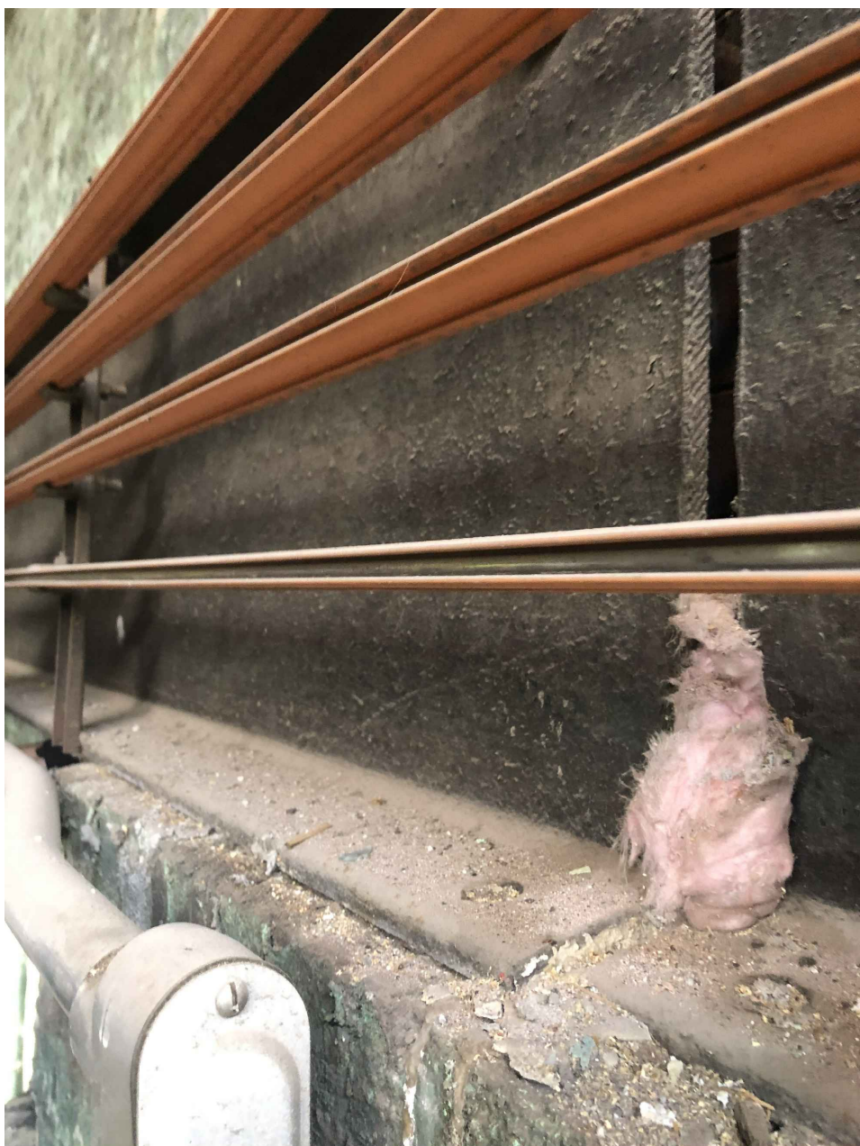
SAMPLE OF ITEM: (G) RUNWAY BEAM SEGMENTS ARE NOT ALIGN WITH ONE ANOTHER
