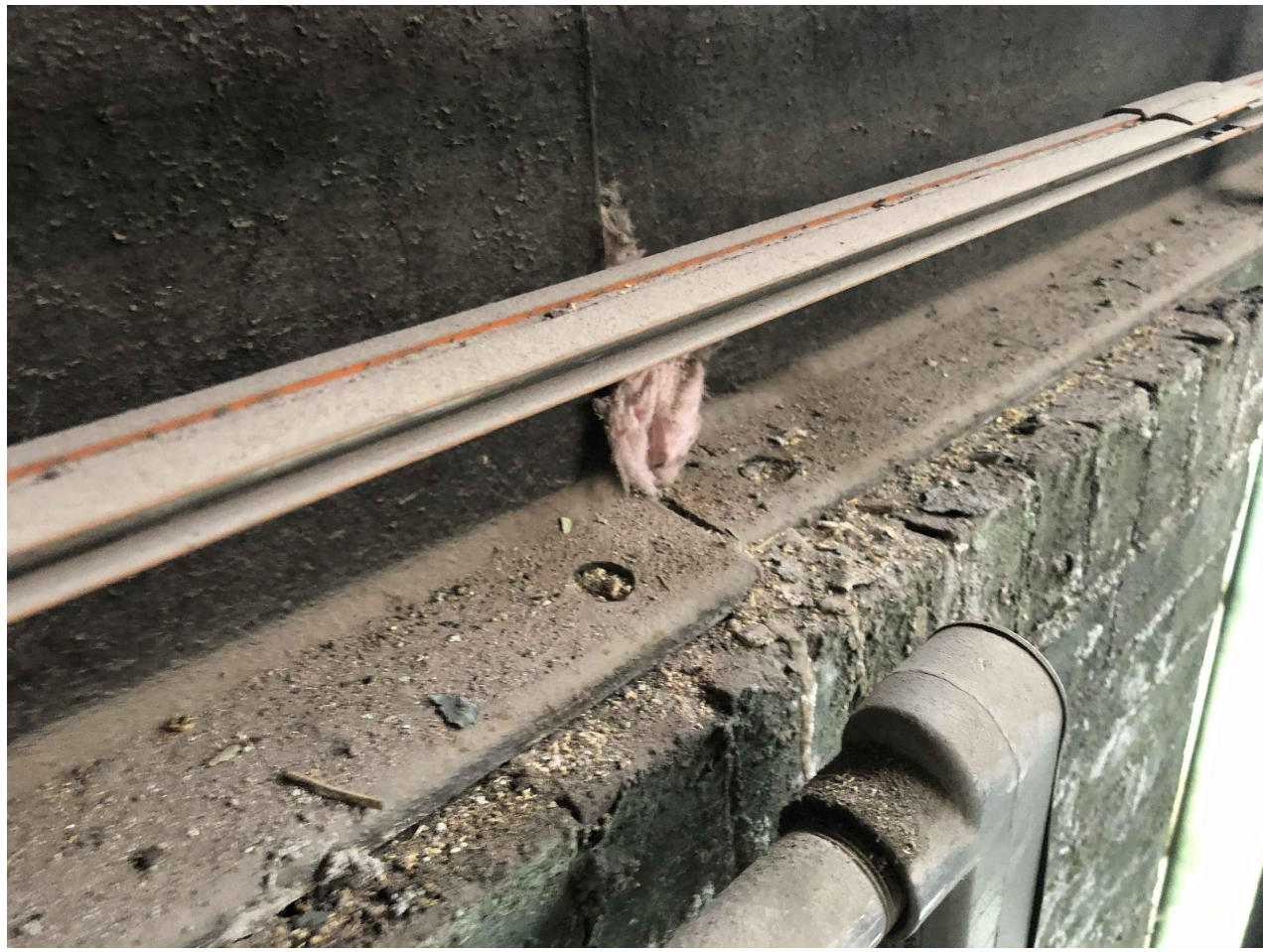
SAMPLE OF ITEM: (E) HOLES IN BOTTOM FLANGE OF THE RUNWAY BEAMS WITH NO ANCHORS
