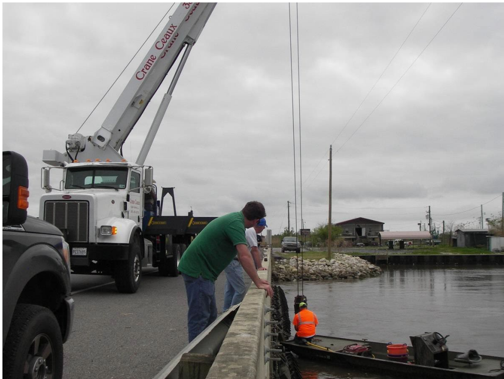
Photo No. 8 - CS-29 Black Bayou Culverts – Lifting Flap Gates for Inspection
