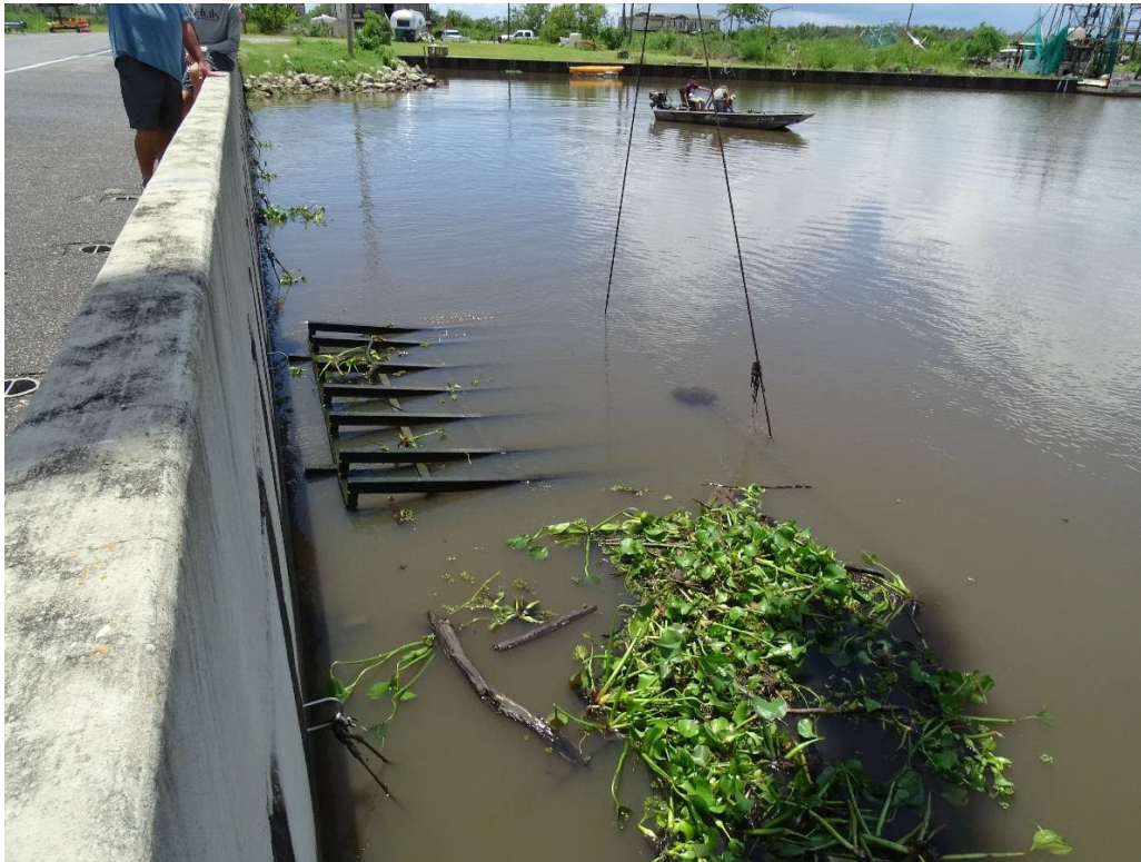
Photo No. 9 - CS-29 Black Bayou Culverts – Lifting Flap Gates for Inspection
