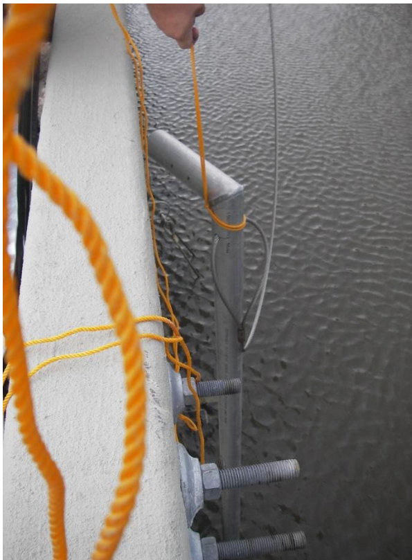
Photo No. 5 - CS-29 Black Bayou Culverts - West Side – Dewatered Flap Gate, Styrofoam Storage Compartments, Cables, Locking Pin Guide Rings, U-bolt in Headwall
