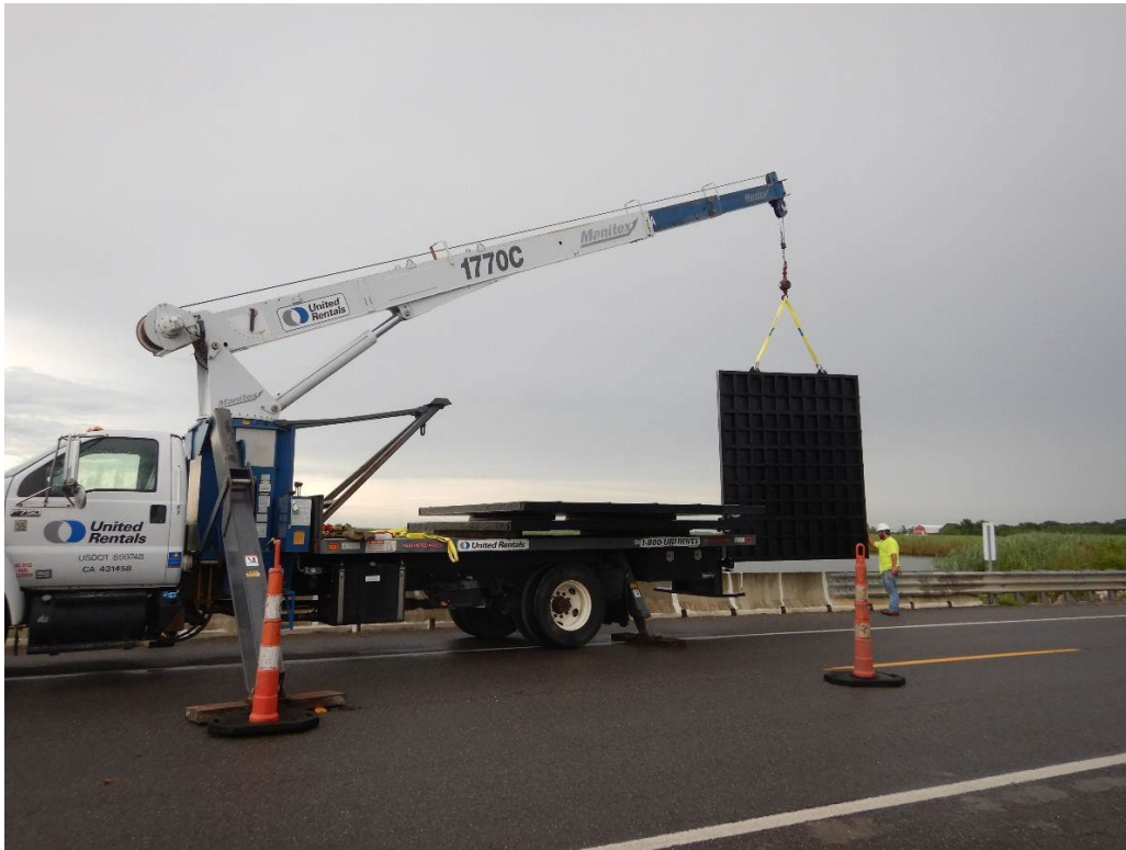
Photo No. 13 - CS-29 Black Bayou Culverts – Installing Sluice Gate for Test Fit
