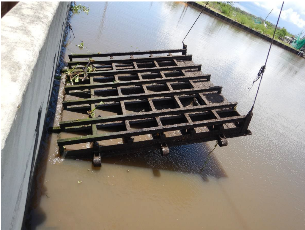
Photo No. 10 - CS-29 Black Bayou Culverts – Lifting Flap Gates for Inspection
