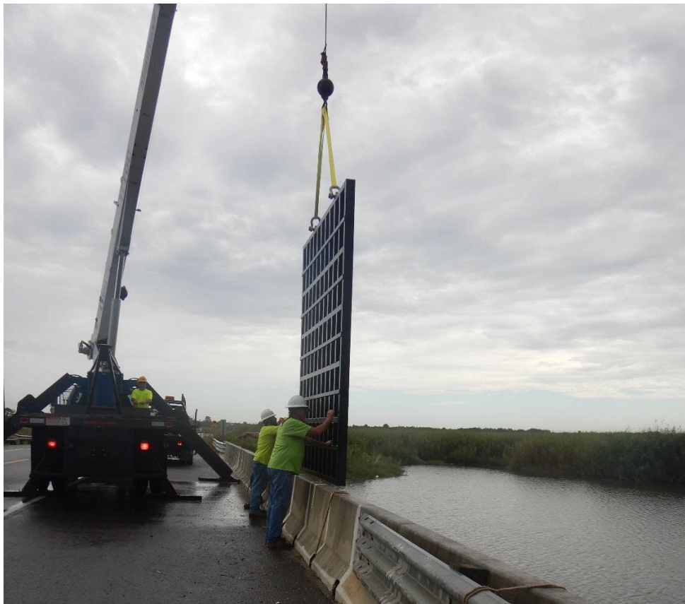
Photo No. 14 - CS-29 Black Bayou Culverts – Installing Sluice Gate for Test Fit
