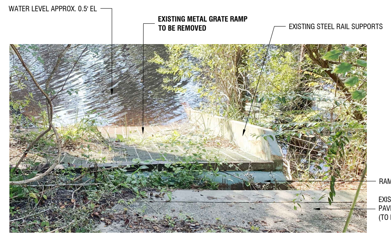
A3 KAYAK LANDING EXISTING CONDITIONS IMAGE NTS
