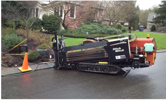
Figure 7.3: Visual of Trenchless -Ground Level Horizontal Boring
