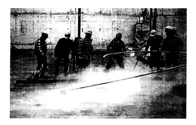
strength development required. Typical addition levels range from 8 to 60 fl oz/100 lbs (520 to 3910 mL/100 kg) of cement, but levels as high as 100 fl oz/100 lbs (6520 mL/100 kg) of cement can be used. For freeze protection purposes typical addition rates are between 60 to 80 fl oz/100 lbs (3910 to 5220 mL/100 kg) of cement.
