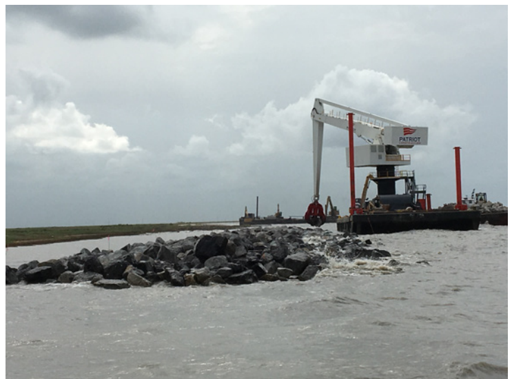
Constructing shoreline protection along the Gulf shoreline of Rockefeller Wildlife Refuge.
