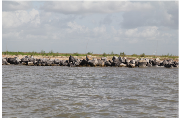
Shoreline protection being constructed along the Rockefeller Wildlife Refuge Gulf shoreline.
