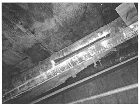
**Photo 8** View of significantly damaged asbestos-containing (60% Chrysotile) White Pipe TSI under floor deck.
