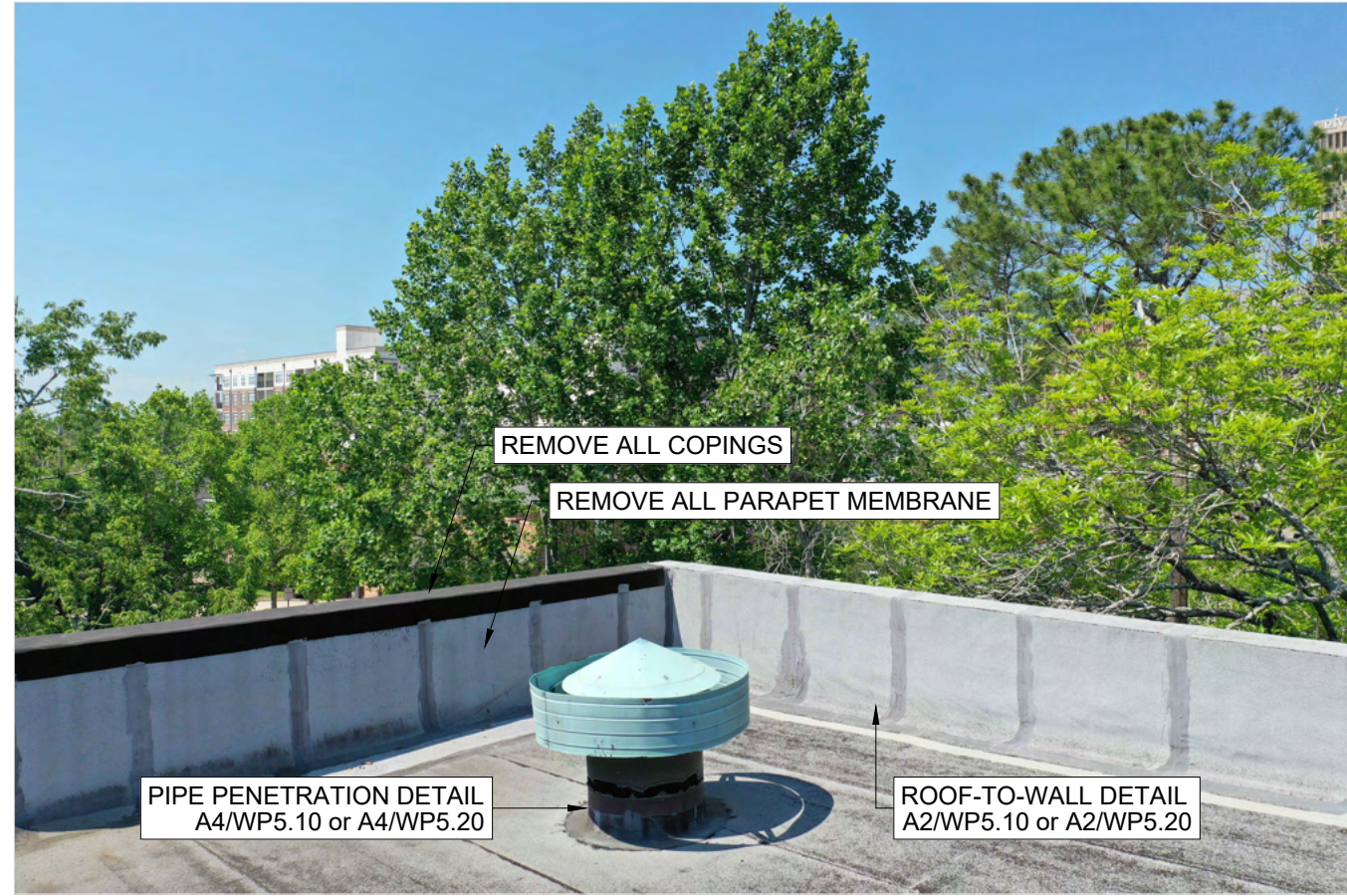
B3 PARAPET COPING TO BE REMOVED G0.01 SCALE: NONE ARCH REF: NONE
