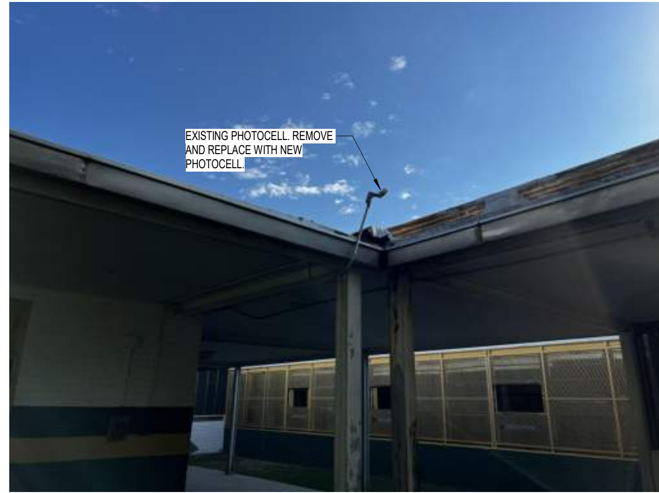
4 PHOTO 4 - CANOPY MOUNTED PHOTOCCELL N.T.S.
