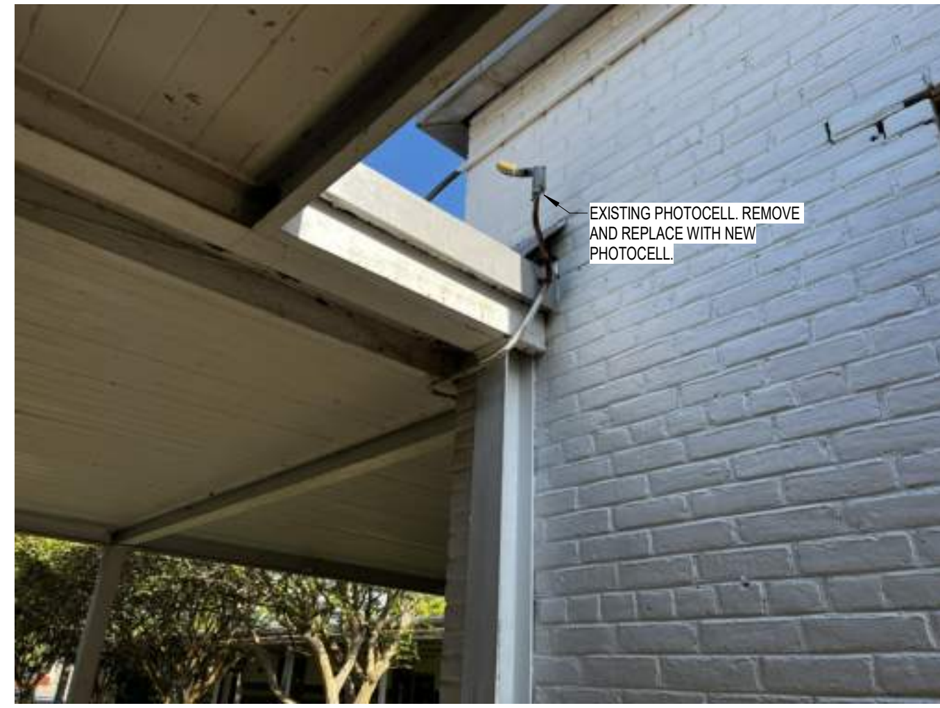
1 PHOTO 1 - CANOPY MOUNTED PHOTOCCELL N.T.S.
