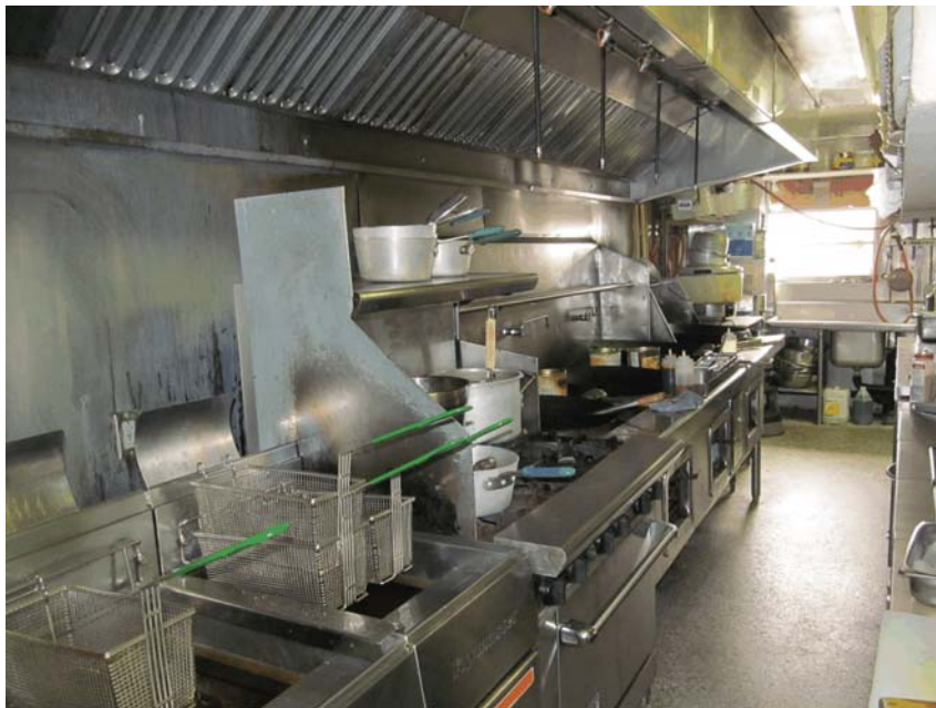
8. Food preparation and cooking area in rear of building. The fire suppression hood system can be seen in upper section of photo.
