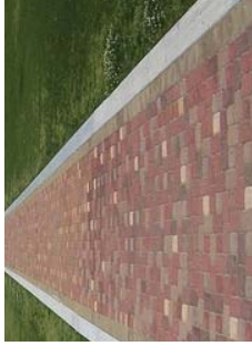
Cox Communications (top) LSU union (middle) LSU pavers (bottom)
